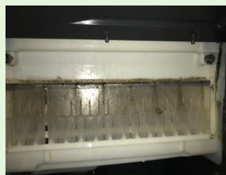
Left: Ice Machine fixed curtain, requiring cleaning, including along the top where a scum line has appeared.
