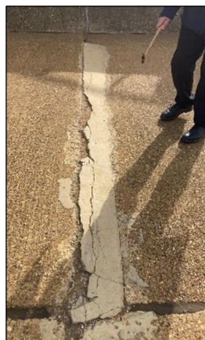
Concrete repair to promenade
