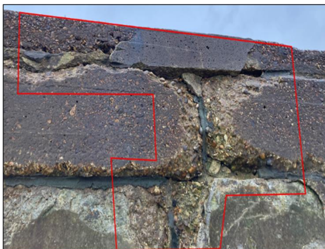
Concrete repair to blockwork seawall
