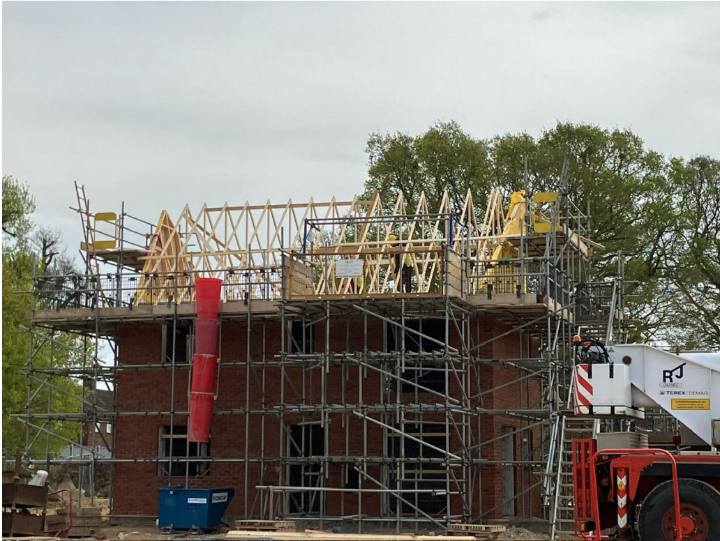
Show home in progress
