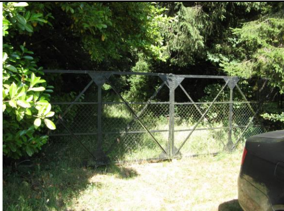
Photograph 1. The main entrance.
