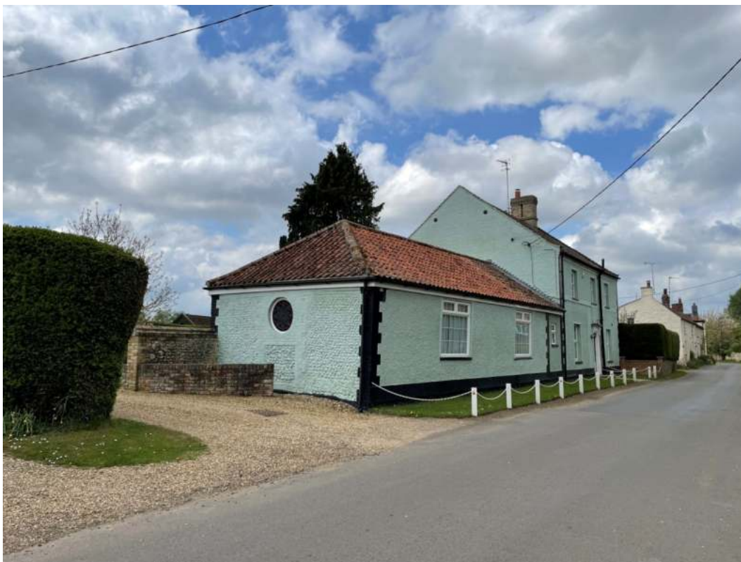
Figure 58: Lattice House, Back Street, circa 1750
