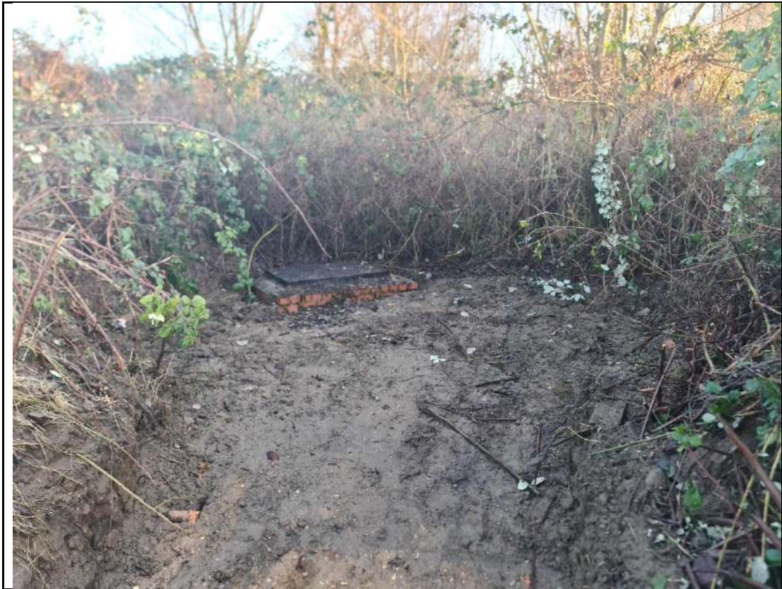
Photograph 7: drain cover and area cleared
