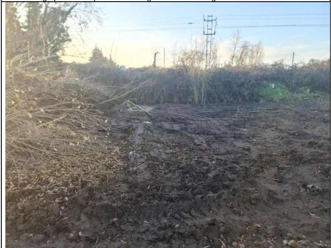
Photograph 6: Cleared area and access cover next to drain.
