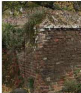
Red brick wall
