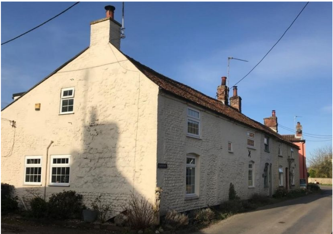
Figure 21: Row of buildings between Latitat Cottage and Sunshine Cottage
