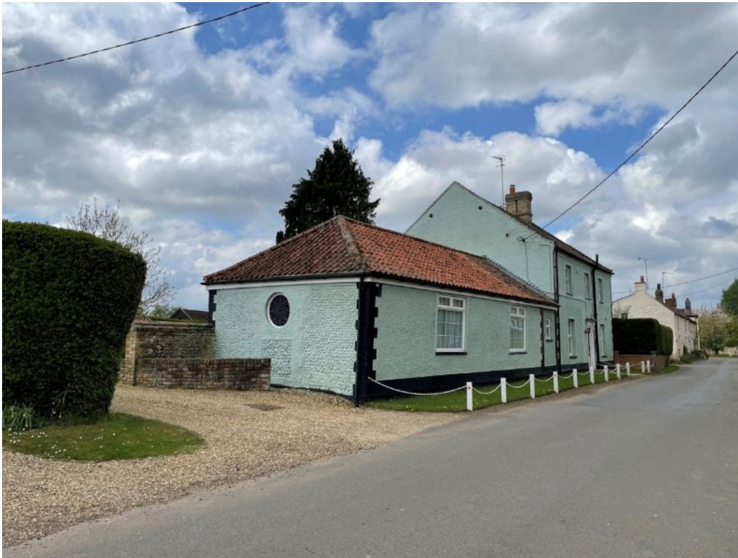
Figure 58: Lattice House, Back Street, circa 1750
