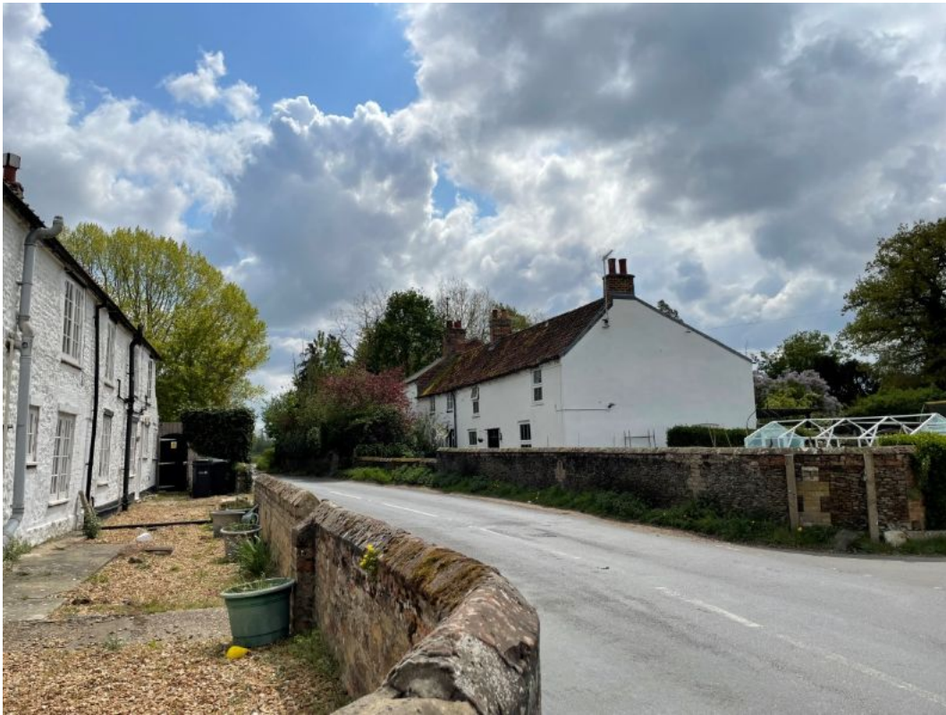
Figure 60: Cluster of Estate Cottages, East Walton Road and Back Street circa mid 1800's (B1153)
