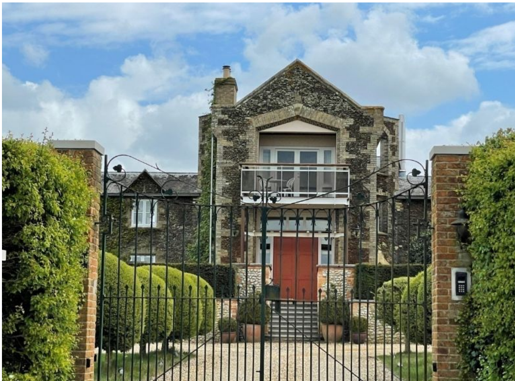
Figure 65: Eastgate House, Front façade.
