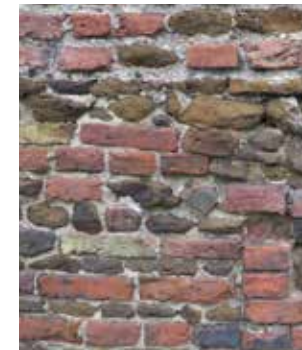
Red brick and carstone boundary wall
