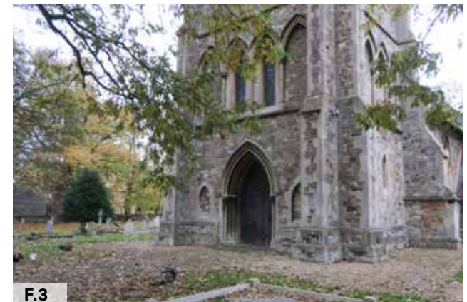
Figure 03: West tower of Grade-II listed All Saints Church (NHLE 1342413)
