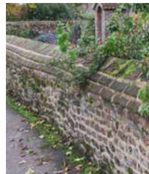
Red brick wall
