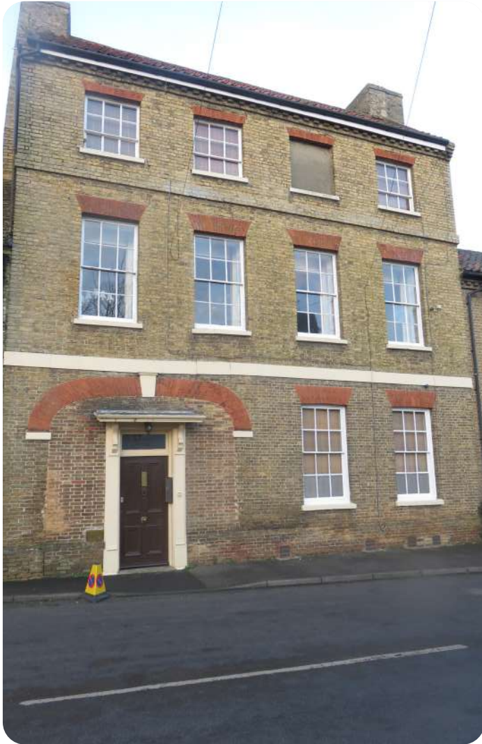
Figure 150: The house immediately east of All Saints Lodge is a 3-storey building made of gault brick with plain tile roof and original sash windows
