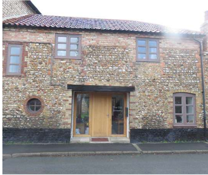
Figure 41: The old Brewery with its contemporary door on Oxborough Rd
