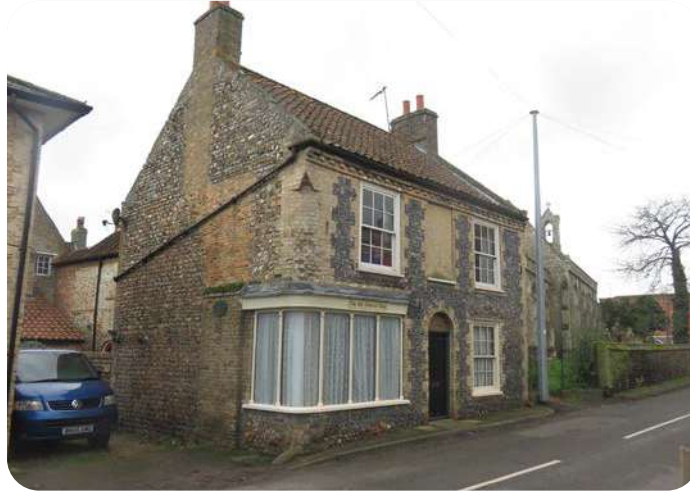
Figure 147: The Old Chemist Shop (1824) is a two storey listed building of flint with gault brick, pantiled roof and shop windows on the ground floor
