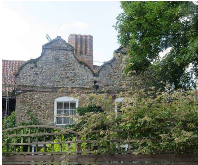
Figure 18: Distinctive use of materials on side gable
