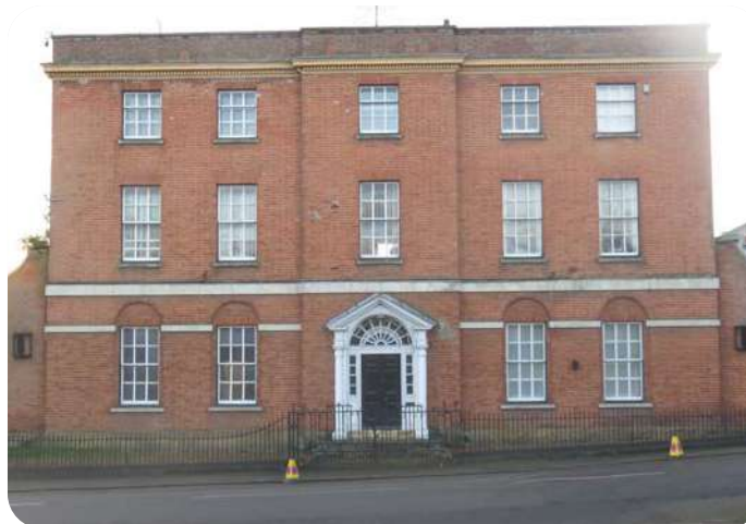
Figure 157: Panelled central door set within door case comprising pair of Tuscan columns and original sash windows
