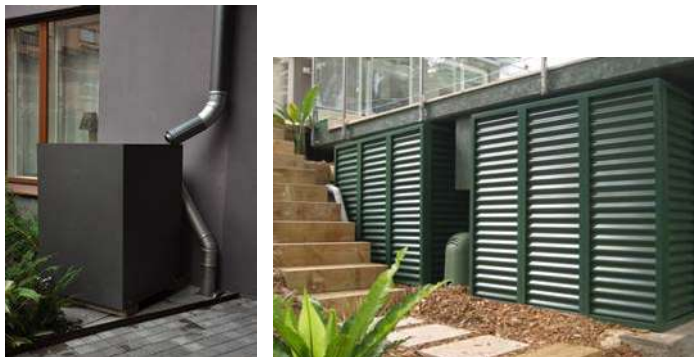
Figure 166: Examples of SuDS designed as a public amenity and fully integrated into the design of the public realm in Stockholm, Sweden
