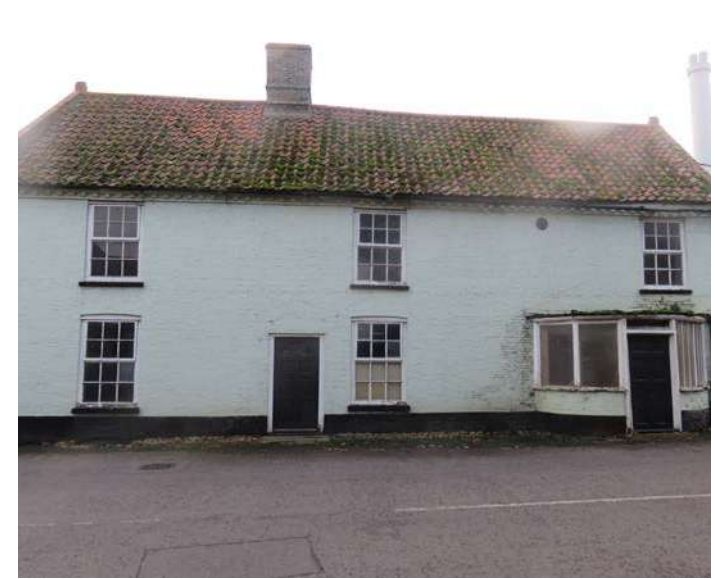
Figure 16: Sash windows are a key feature of the historic core
