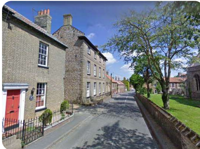
Figure 129: Listed building with front doors and windows facing the High St creating strong sense of safety
