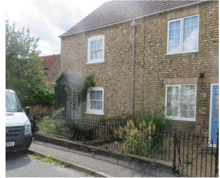
Figure 42: Distinctive and attractive porch
