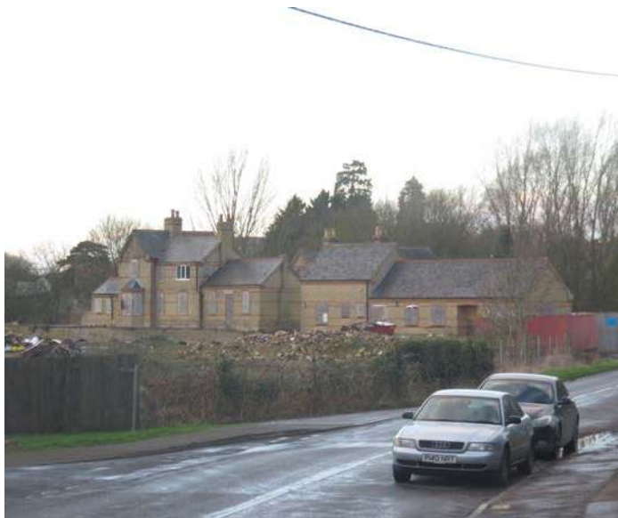
Figure 36: The old station yard - varied roofscape creates visual interest
