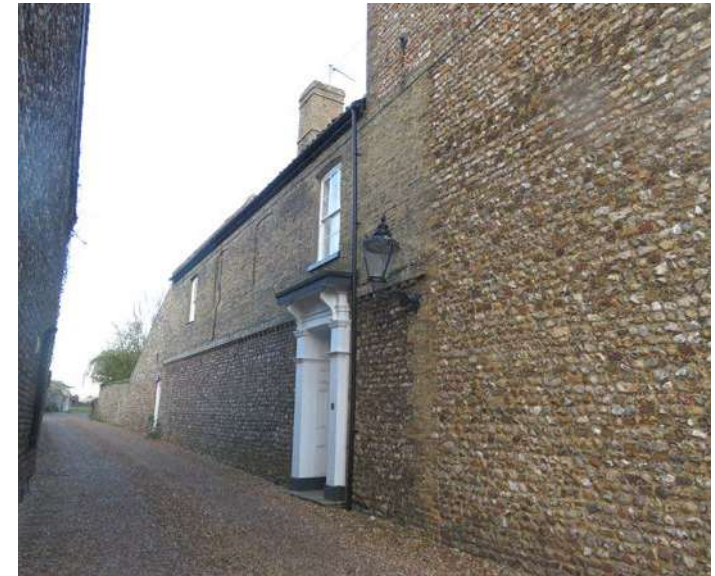
Figure 19: Side passage with flint wall
