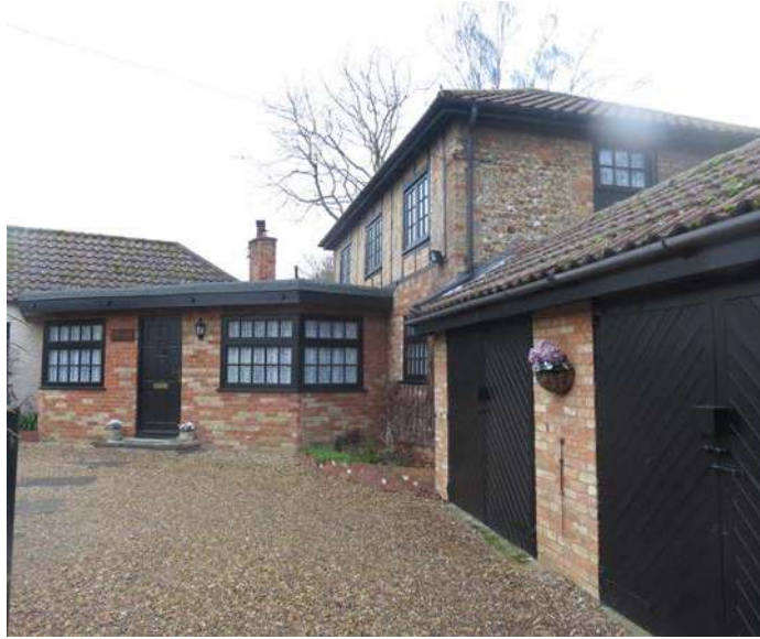
Figure 47: Modern property with single storey extension (The Granary)
