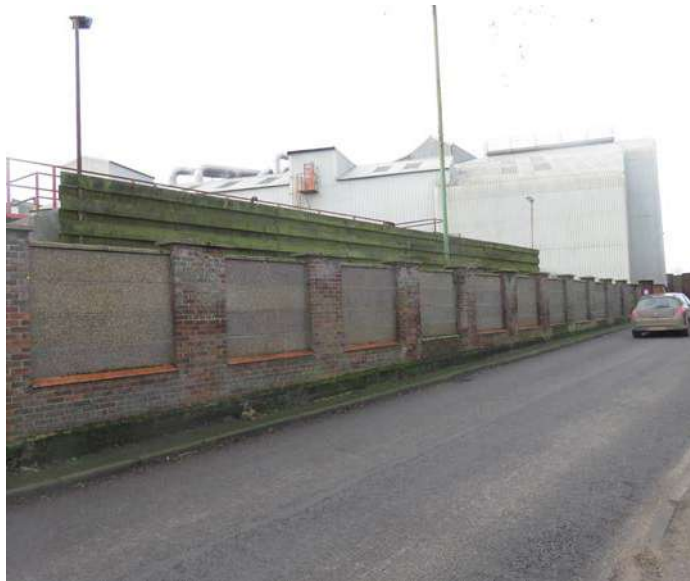
Figure 72: Inactive wall creates a break in the built form of the village here
