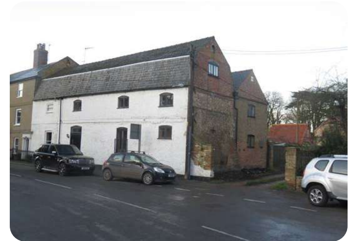
Figure 114: On-street car parking on High Street by the Old Granary
