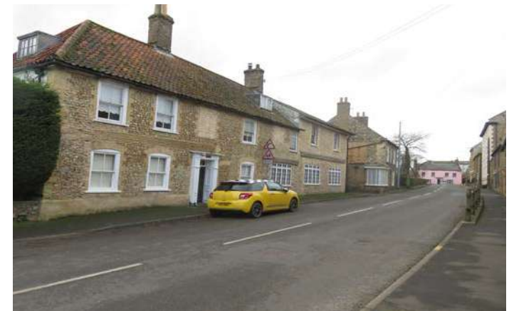
Figure 3: View of High Street in historic core of the village
