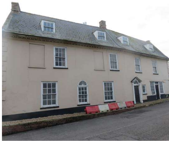
Figure 15: Varied facade showing use of sash windows
