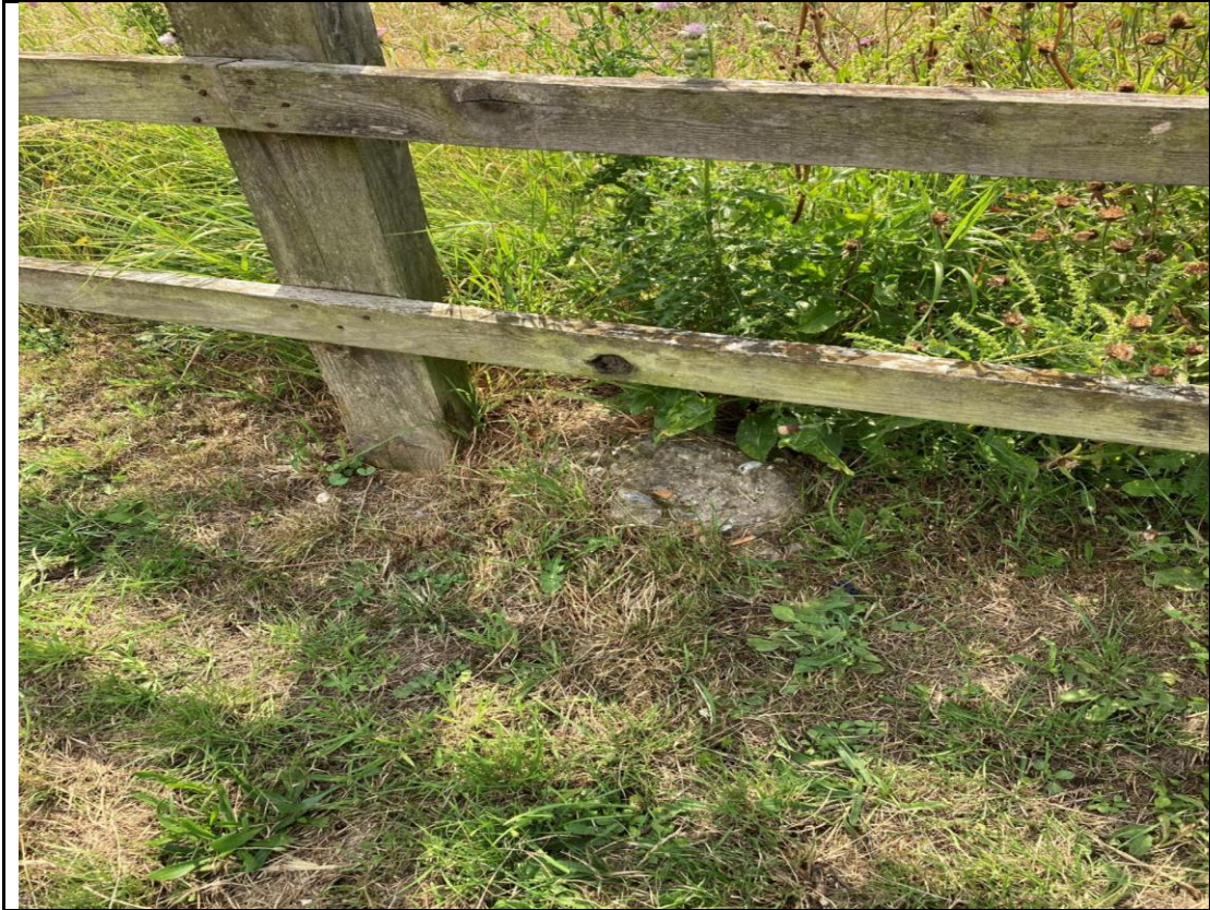
Photograph 7: Buried concrete close to fence
