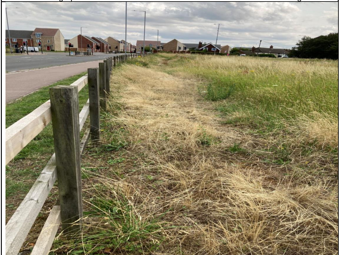
Photograph 6: Remnant hardstanding, effect on vegetation growth
