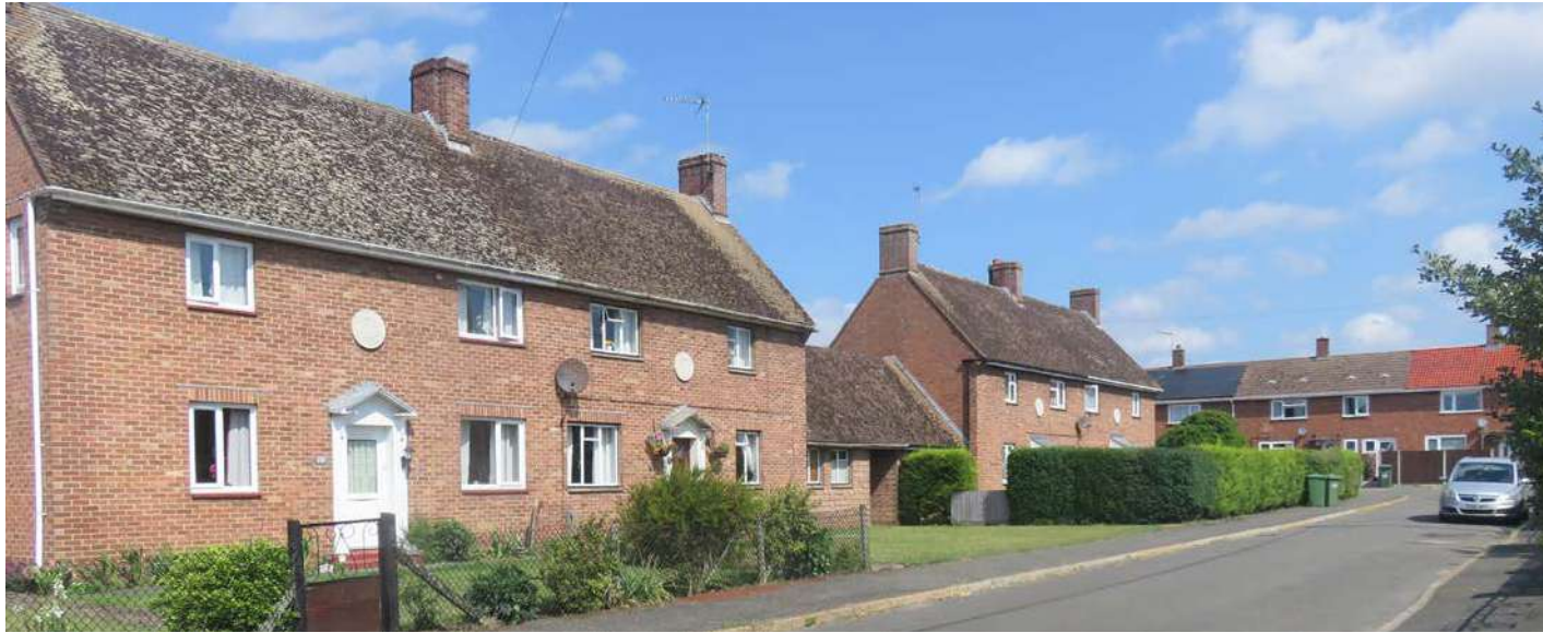
Figure 66: Buckenham Drive is the oldest estate in the village (1945) and creates strong character and sense of community
