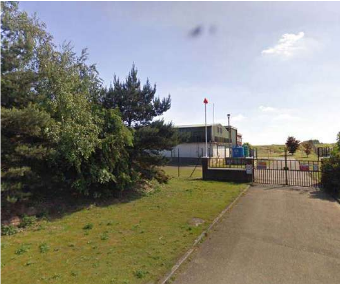
Figure 91: Stoke Ferry Anglian Water Treatment Works
