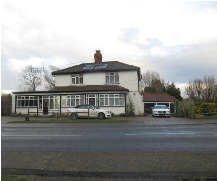
Figure 27: The former Old Bull public house on Bridge Road
