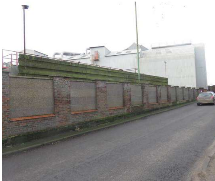
Figure 72: Inactive wall creates a break in the built form of the village here
