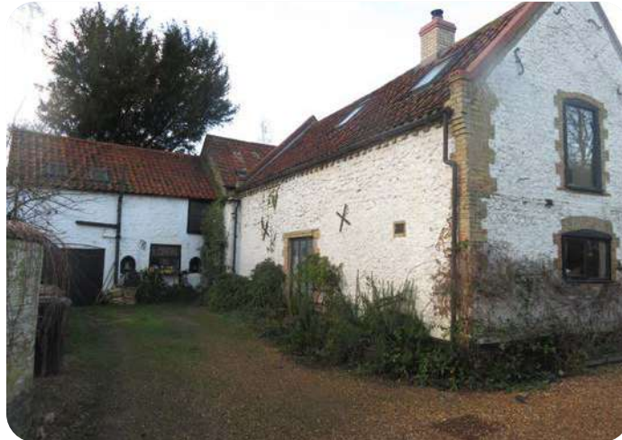
Figure 152: Good example of brick quoins at the corner of Coachman's Cottage
