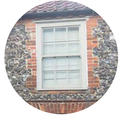
MASONRY WORK AROUND WINDOWS
