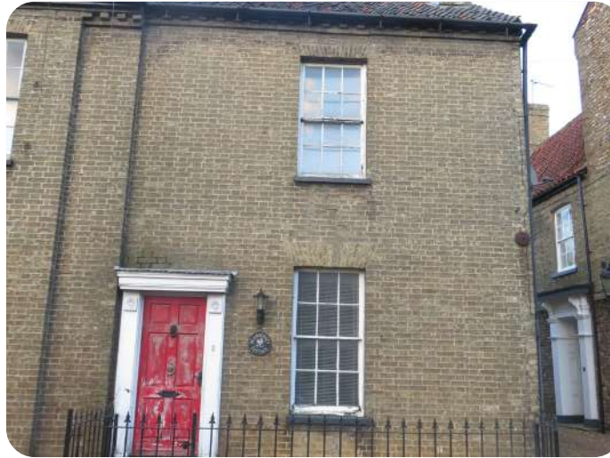
Figure 160: Original Sash windows vertically aligned on Deans Croft Cottage facade
