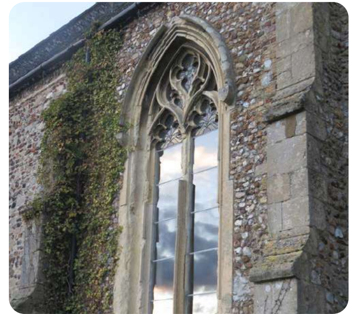
Figure 151: A tall and narrow lancet window with a pointed arch and decoration at its top on one of the All Saints' Church façades
