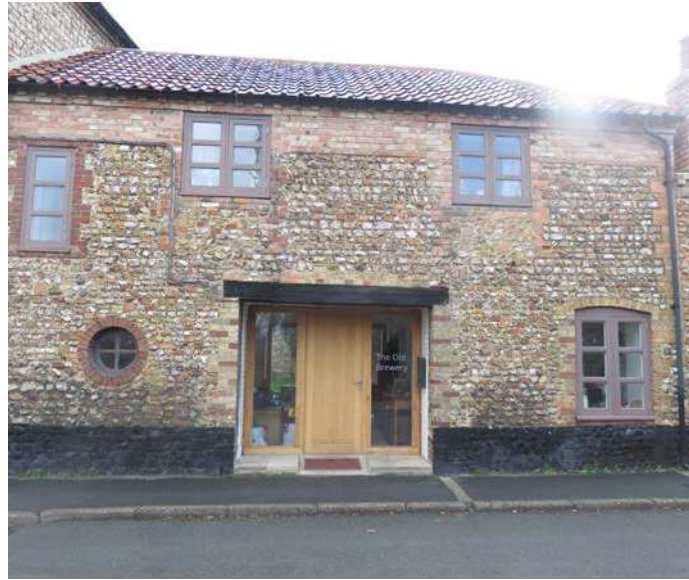
Figure 41: The old Brewery with its contemporary door on Oxborough Rd
