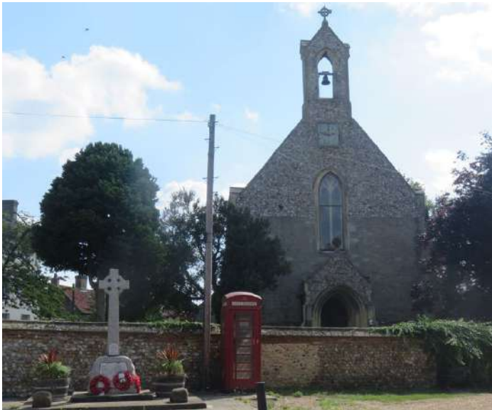
Figure 23: Grade II listed All Saints Church (now privately owned)
