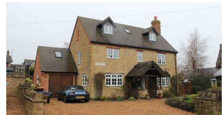
Figure 161: Good example of side extension (garage). The addition to the new part respects the building's mass character and roofline
