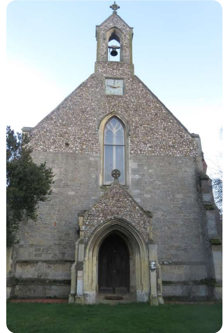
Figure 146: The Church of All Saints located by the Hill is a landmark built of ashlar, clunch and flint with slate roofs.
