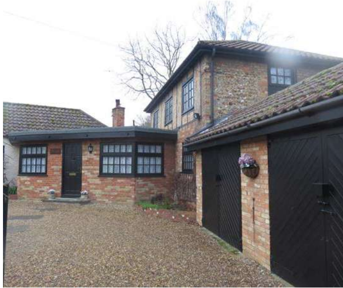
Figure 47: Modern property with single storey extension (The Granary)
