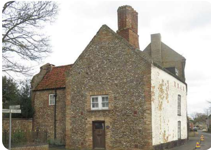
Figure 148: The Old Saints Lodge and Crown House have unusual Elizabethan cylindrical chimneys. The Old Crown also has ornate gables in Dutch Baroque style, which are unusual for West Norfolk
