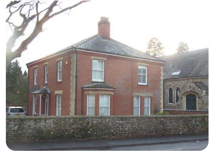
Figure 159: Door left, with distinctive iron pillars carrying flat entablature with scalloped slates. Bay window to side elevation
