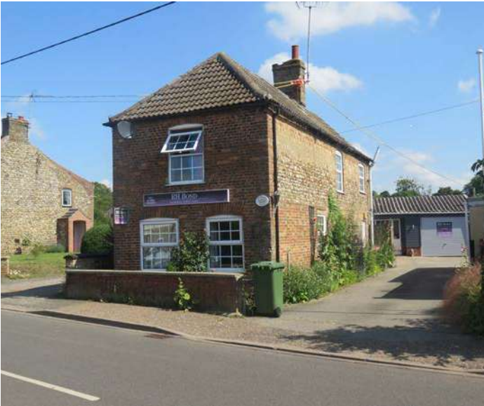
Figure 58: Older property with pantile roof
