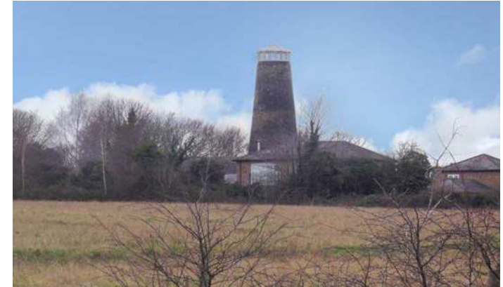
Figure 1: Grade II listed Tower Mill
