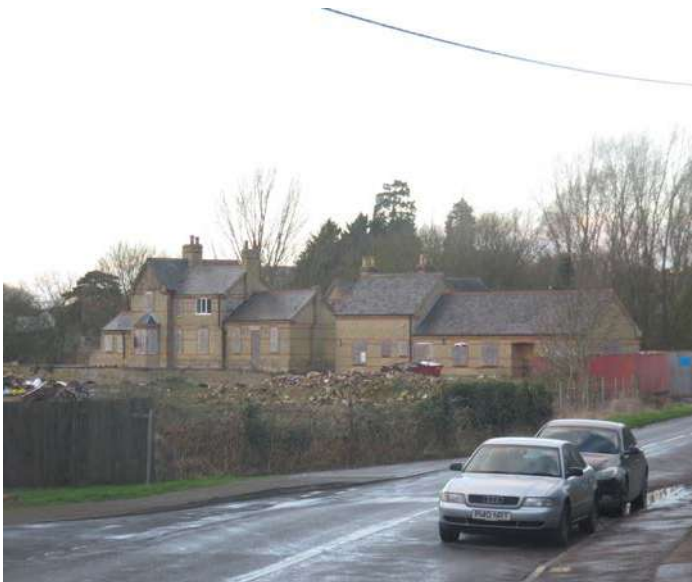
Figure 36: The old station yard - varied roofscape creates visual interest
