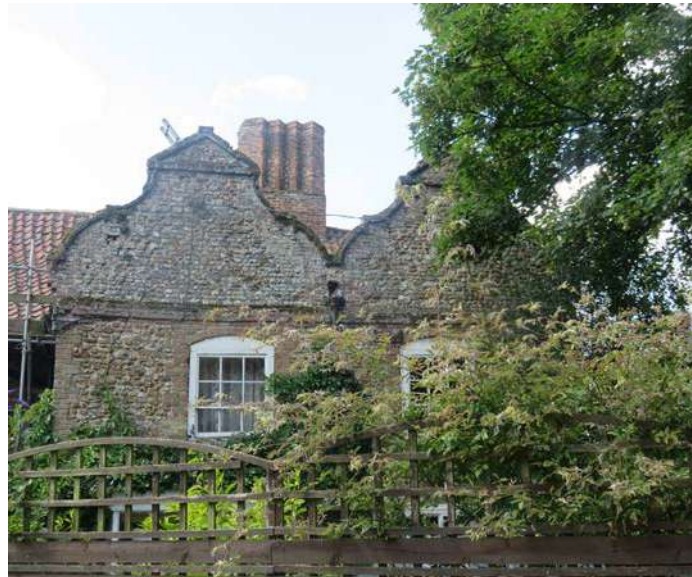
Figure 18: Distinctive use of materials on side gable
