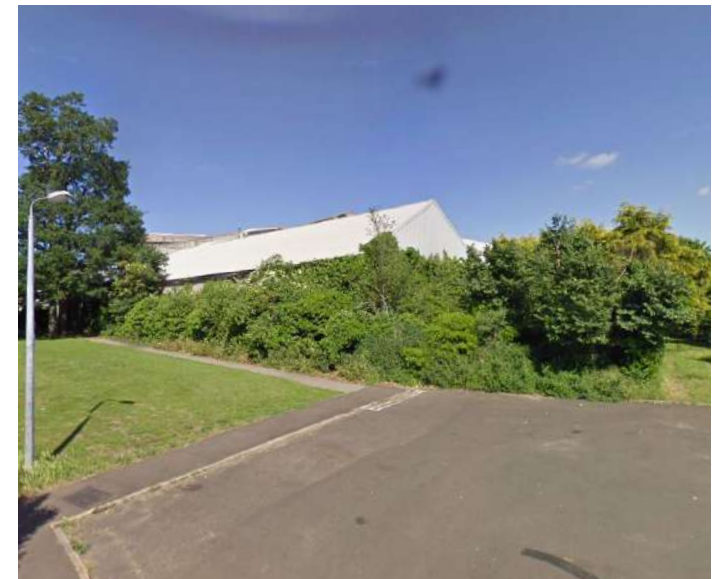
Figure 73: Tall industrial structures within the 2Agriculture site visible from Buckenham Drive
