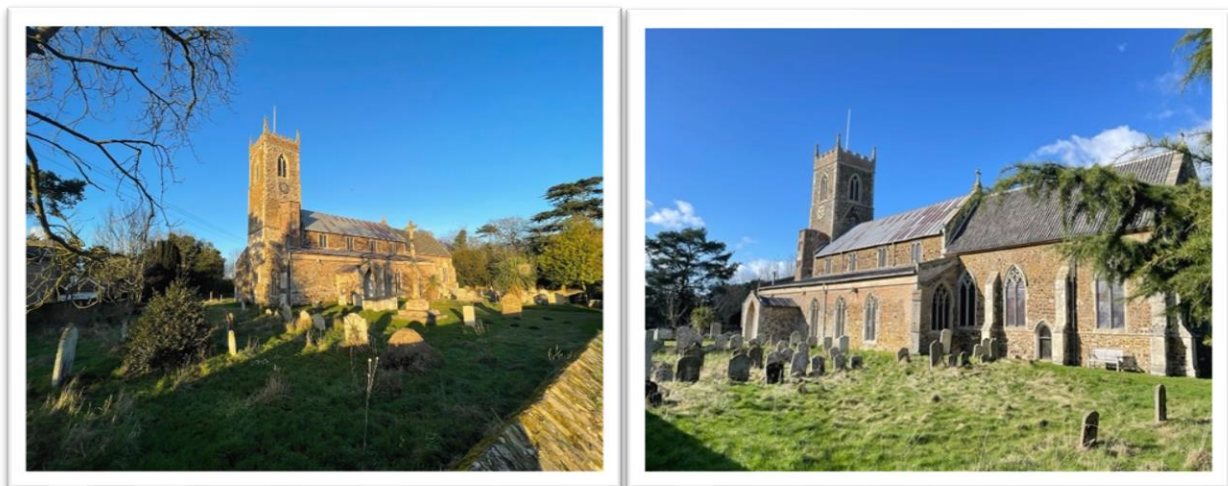
Figure 17-Pictures of the St Peter and St Paul's Church
