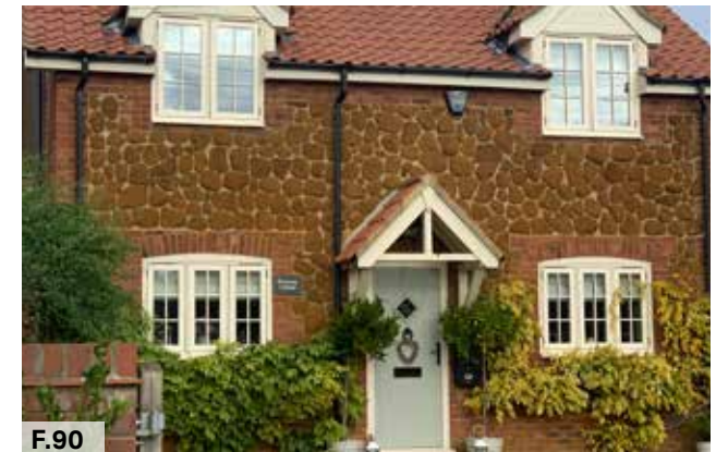
Figure 90: Contemporary building using traditional local materials - carstone, red bricks, and clay pantiles
