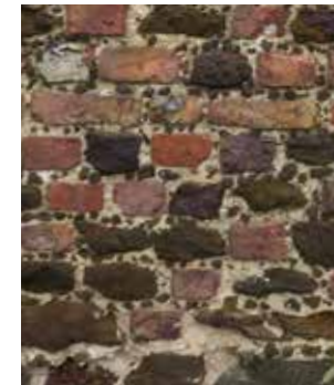
Red brick and carstone boundary wall with galletting
