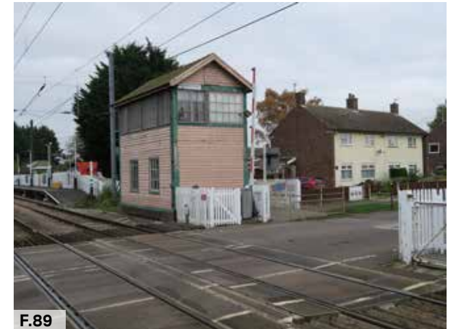
Figure 89: Railway building serving as an informal landmark and gateway at the edge of the settlement
