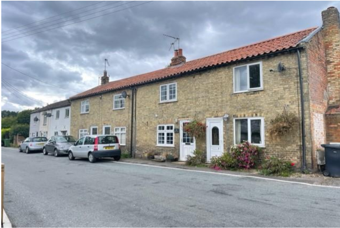
Two rows of Victorian terraced cottages, 24-32b and 40-48 Mill Road
