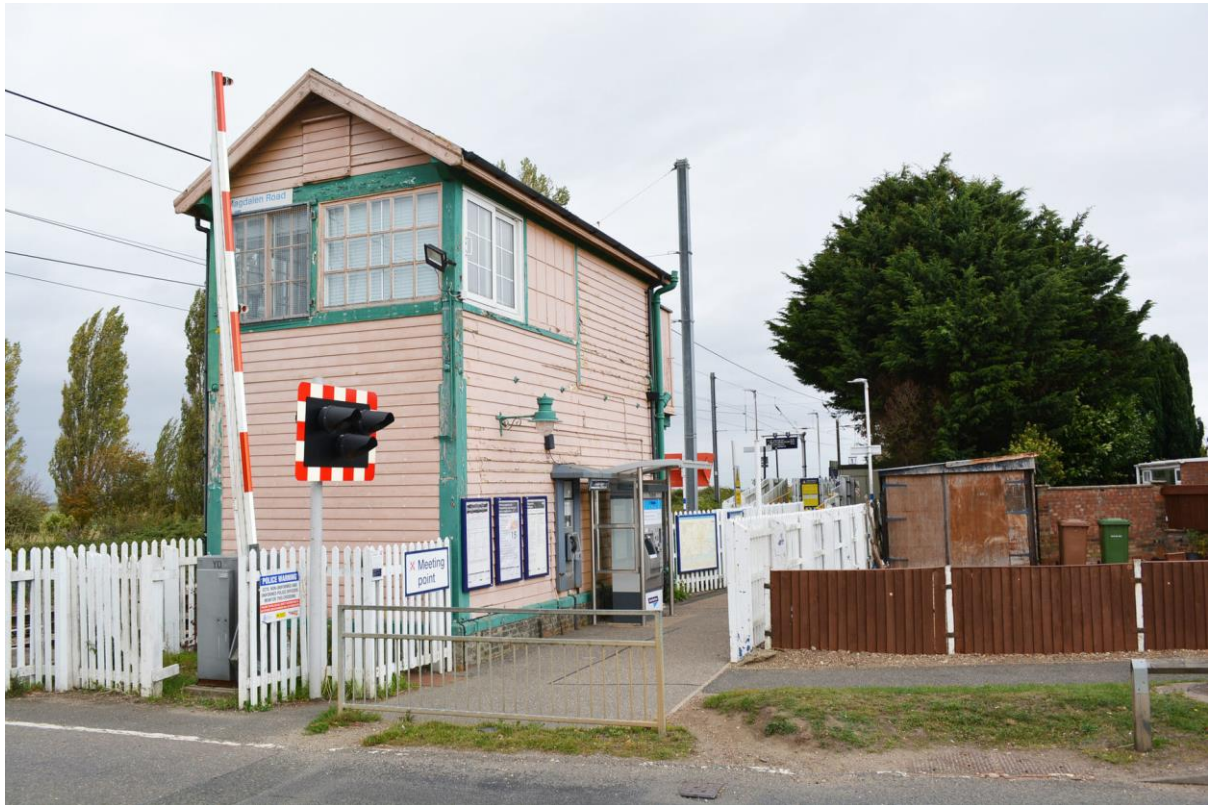
Picture of the entrance into Watlington Railway Station
