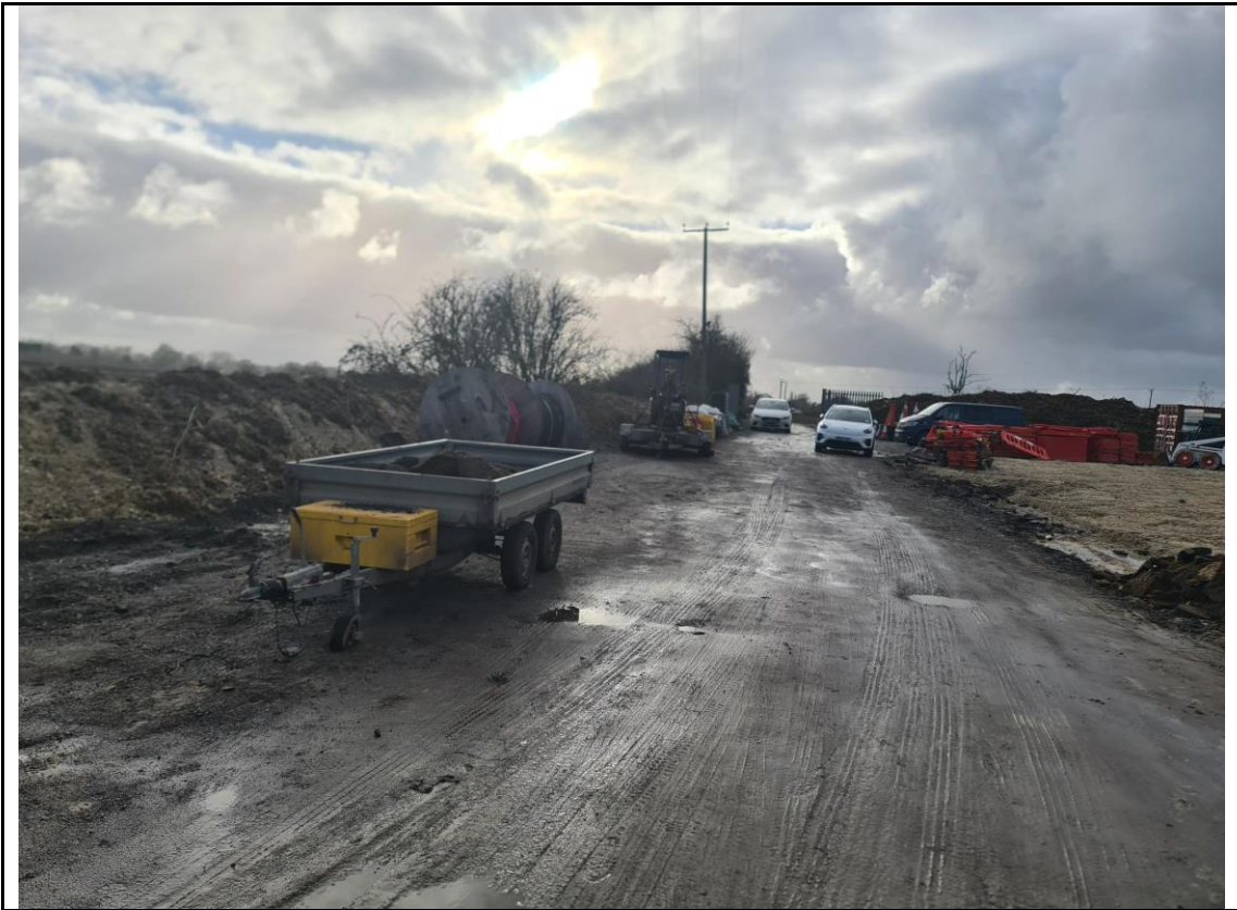
Photograph 47: Parking/storage area showing chalky material used to level site
