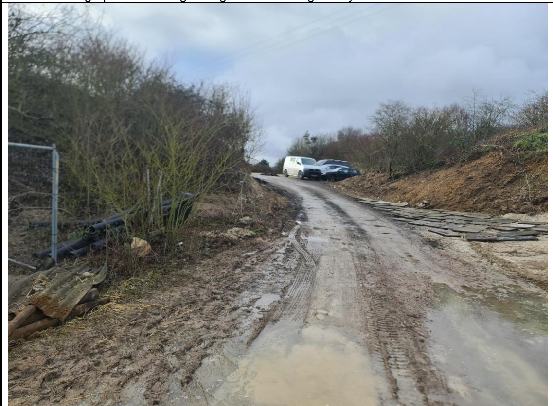
Photograph 48: Track leading into the pit
