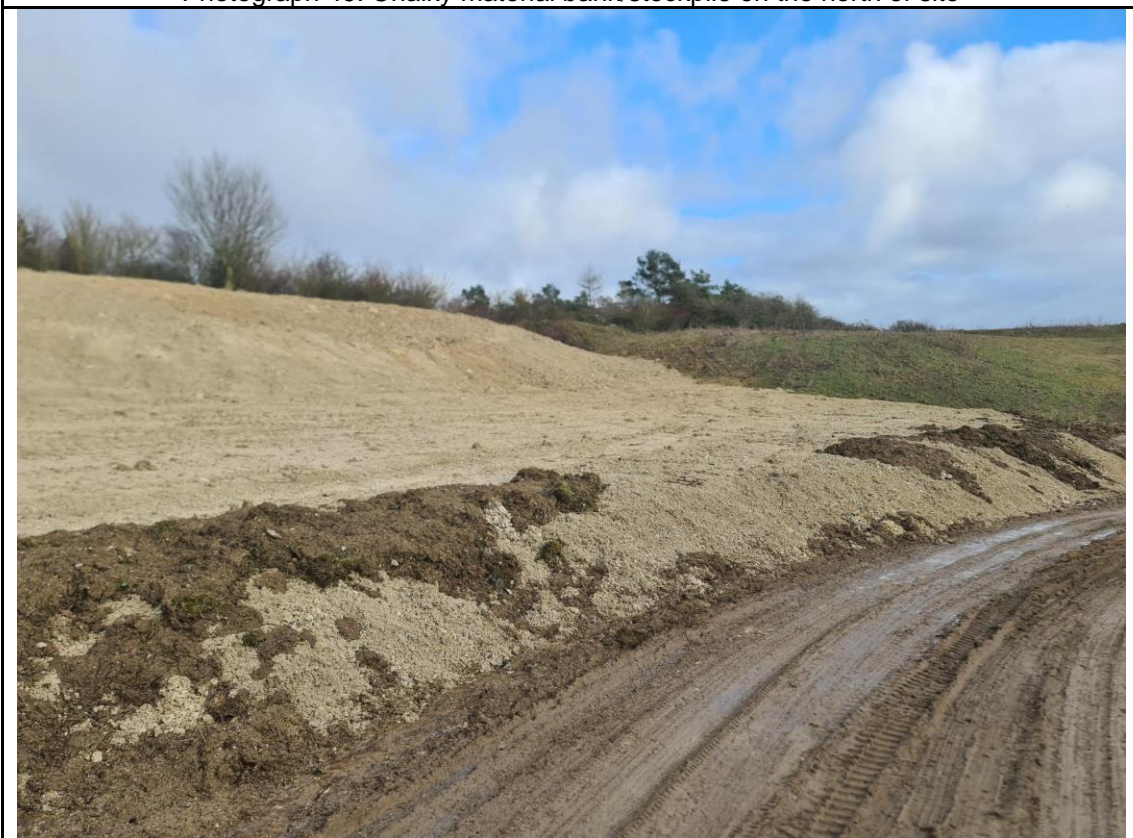
Photograph 50: Chalky material bank/stockpile
