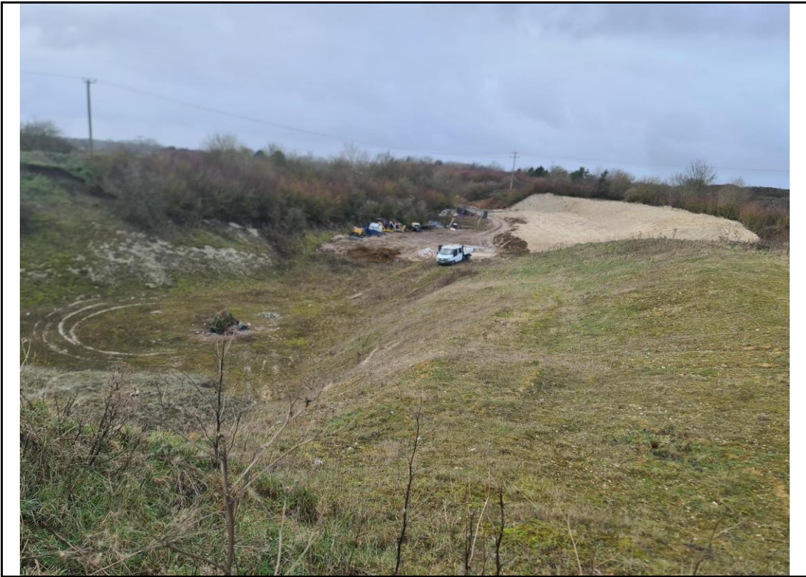
Photograph 45: Pit and track in east of site
