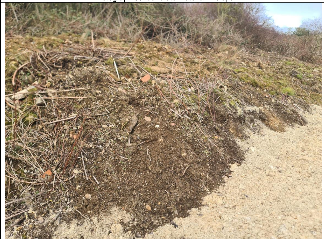
Photograph 56: Soil slope barrier to the western boundary
