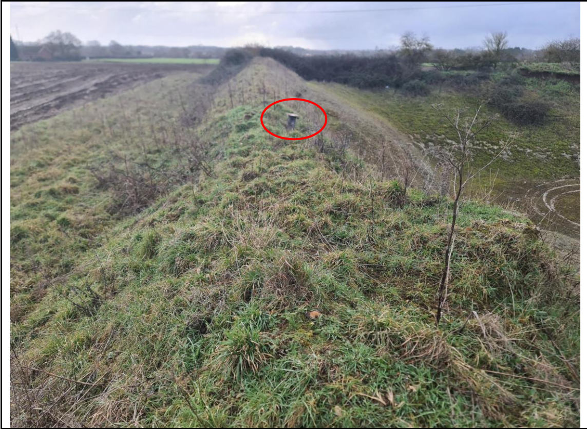
Photograph 43: Bund on the east of site. Borehole present.
