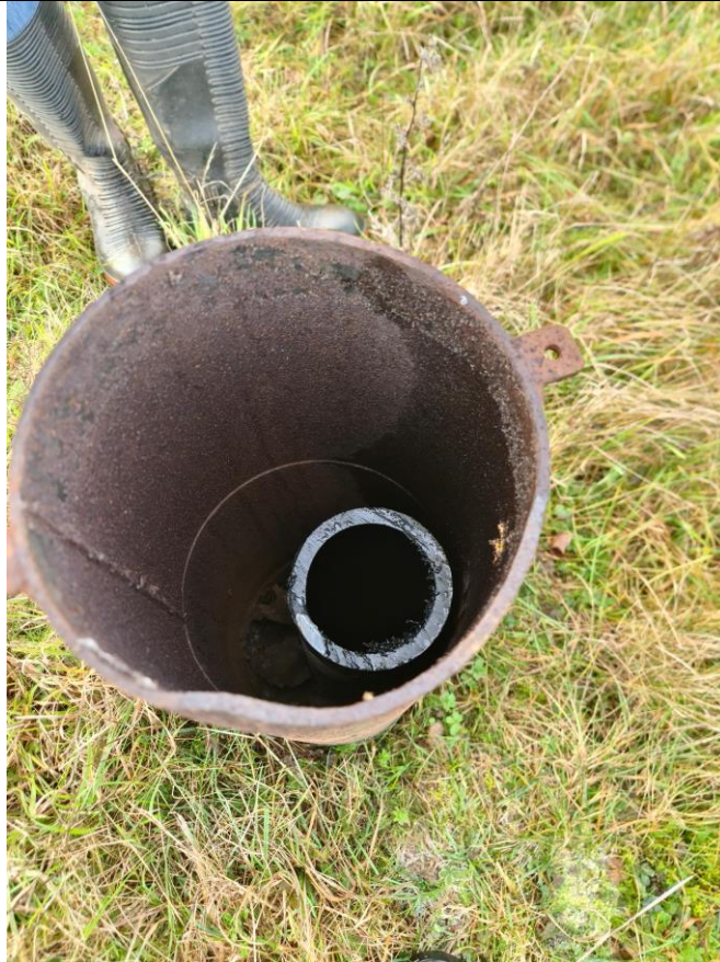
Photograph 26: L2 monitoring borehole, cap removed for photograph)
