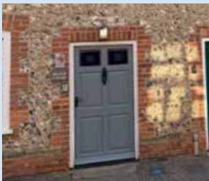
Wooden door with red brick finish
