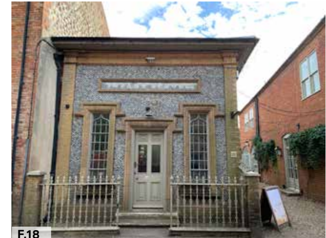
Figure 18: National Westminster Bank, Grade II, built in 19th century with pebble flint, gault dressings, cast iron casements and decorations
