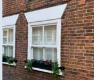
Sash window with lintel above
