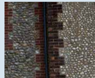
Rusticated brick quoins
