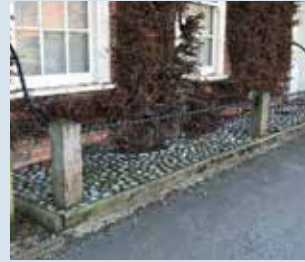
Post with wrought iron metalwork bars
