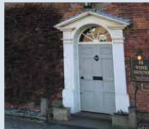
Pedimented doorcase with fanlight
