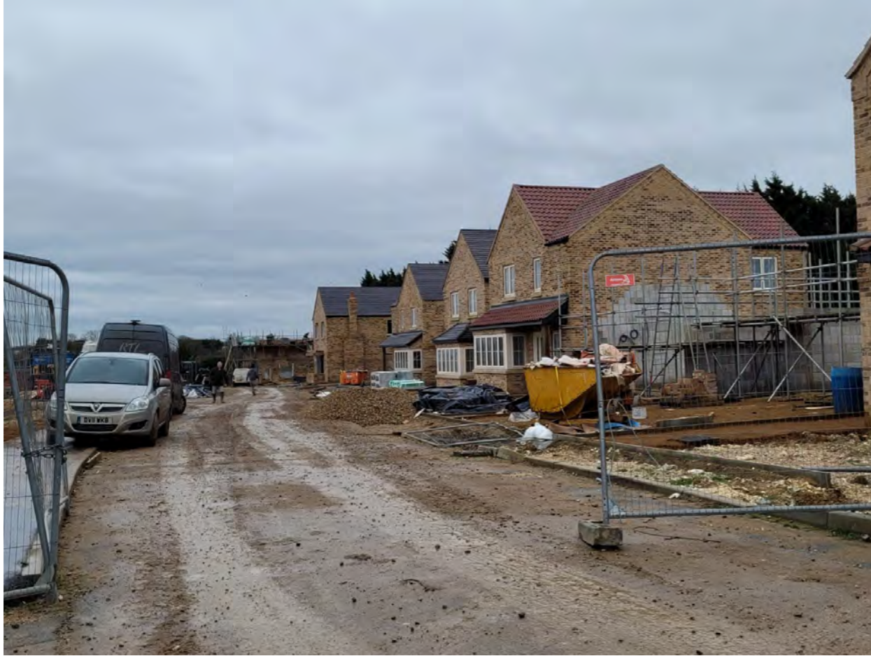
Rear of site still u/c but some watertight
