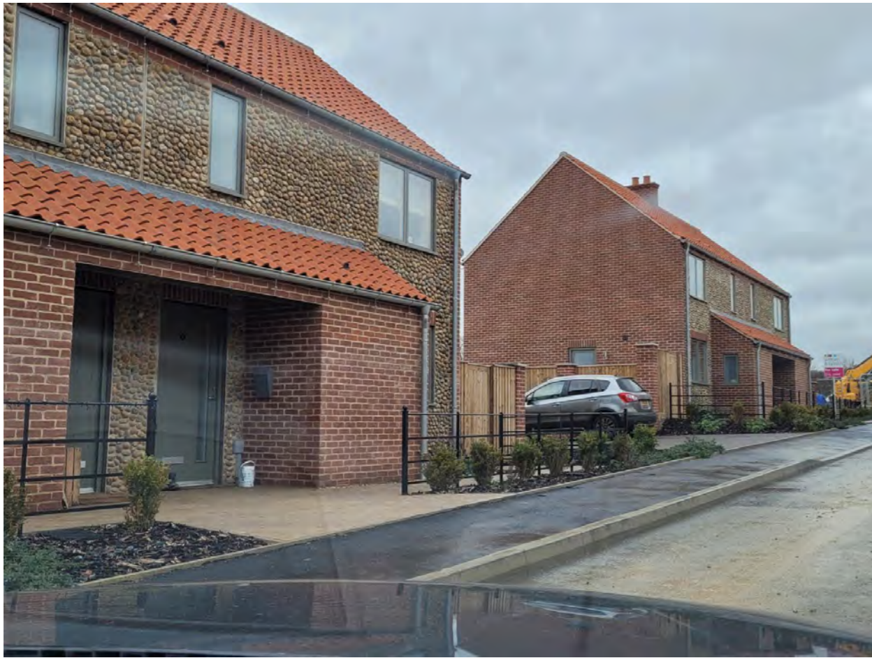
Some close to completion
