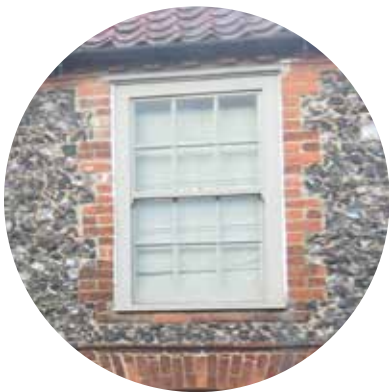
MASONRY WORK AROUND WINDOWS
