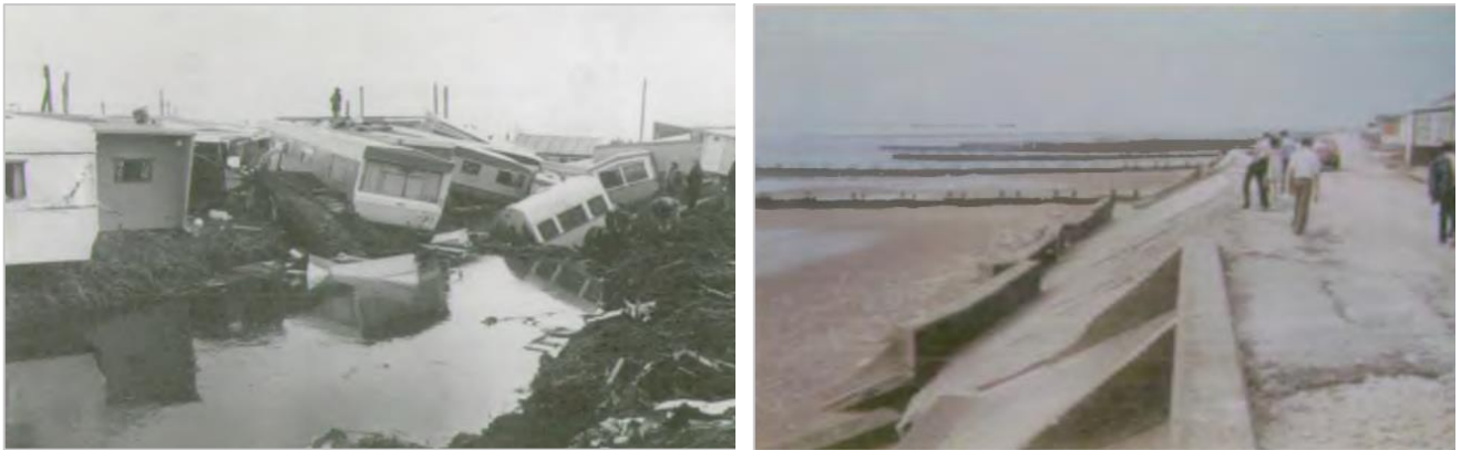
Figure A-19 Damage caused by breach of sea defences at Heacham in 1978. Source: Environment Agency (date unknown, but possibly 1998).
