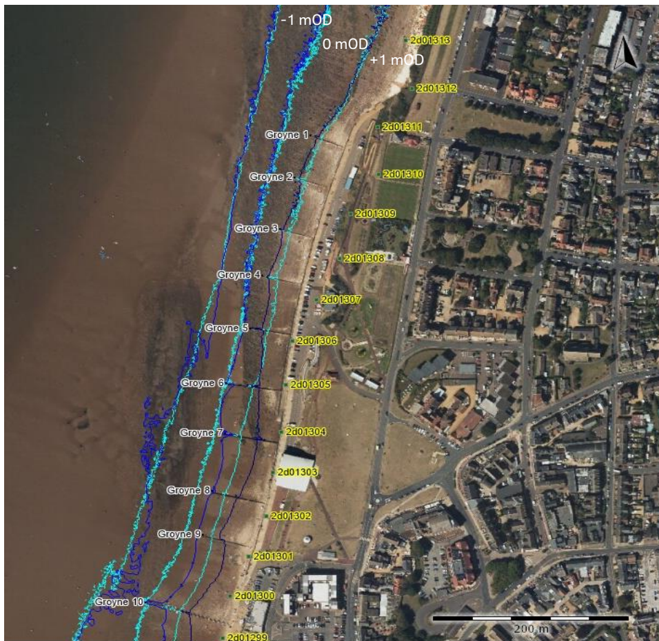
Figure A-25 BCKLWN concrete groyne frontage, with the position of the 0 mOD, +1 mOD and -1 mOD contours generated from 2012 (light blue) and 2020 (blue) LiDAR data. Also shown are the beach transect locations.
