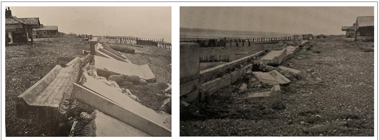
Figure A-16 Damage to Heacham North Beach Wall following 1953 storms, noting the timber groynes that were present at this time. Taken from ICE Conference on the North Sea Floods (1954).
