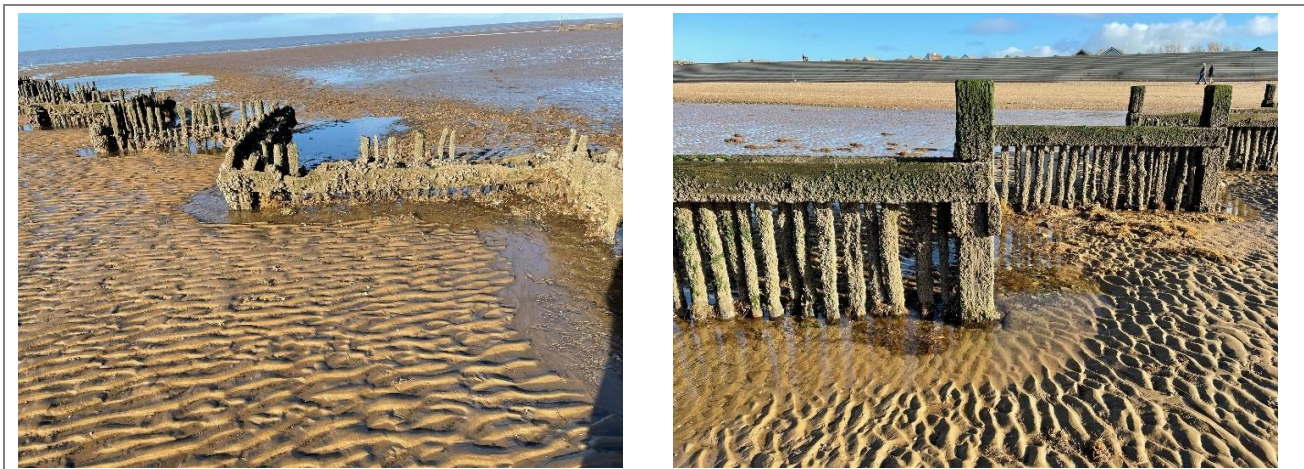
Figure 3-4 Condition of Environment Agency timber groynes.
