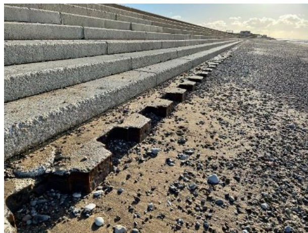
Northern stretch to Groyne EA6
