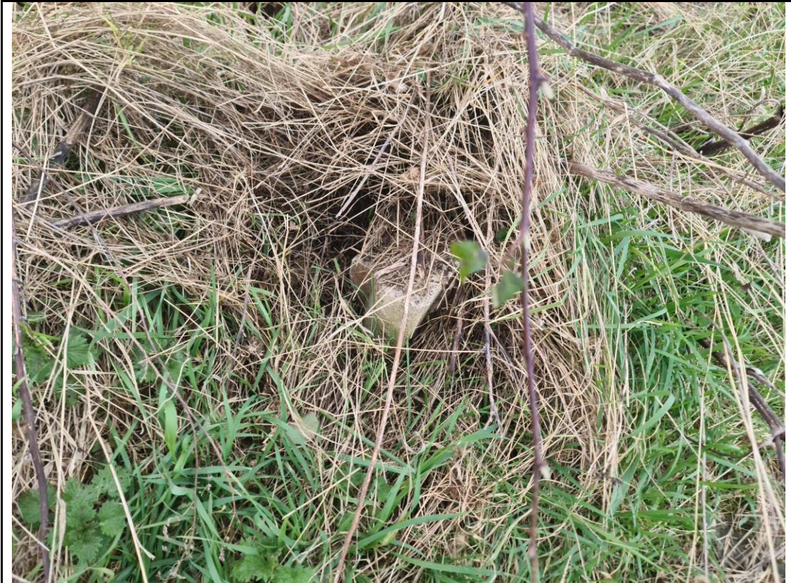
Photograph 7: Lump of concrete exposed at the site surface
