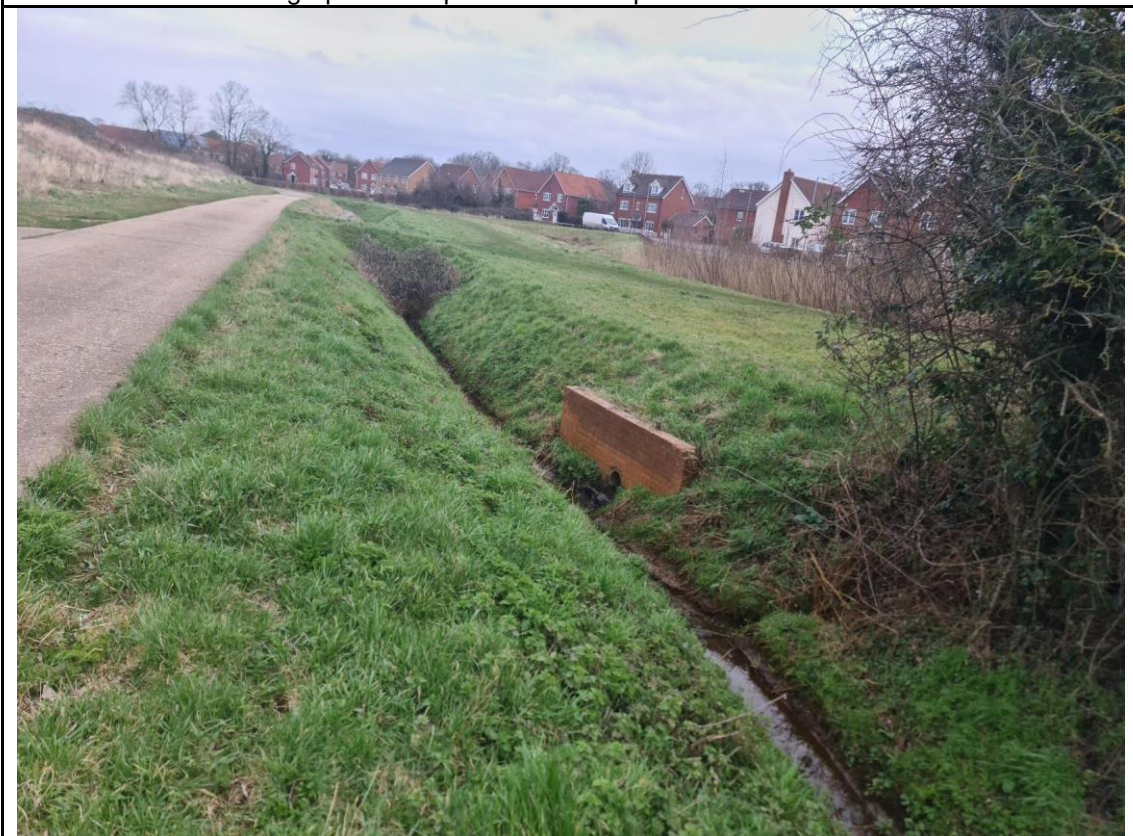
Photograph 8: South portion of the drain running along the east of site. Housing estate in the background showing the proximity to site.
