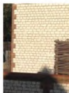
New coursed chalk with brick quoins
