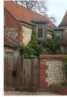
Feature windows finished in grey
