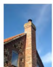
Gable with chimney stack
