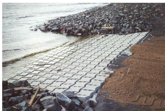
Figure 4-4: Example pre-cast concrete mattress slipway
