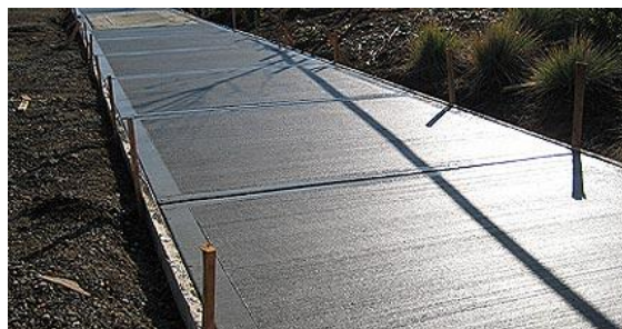
Figure 4-3: Example in-situ poured RC slipway
