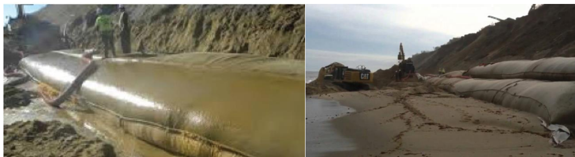
Figure 5-3: Example photographs of sand filled Geotubes in front of steep cliffs
