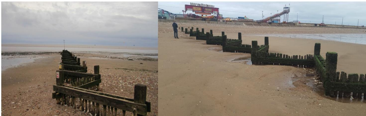
Figure 5-9: Photographs of the timber groynes in Unit B
