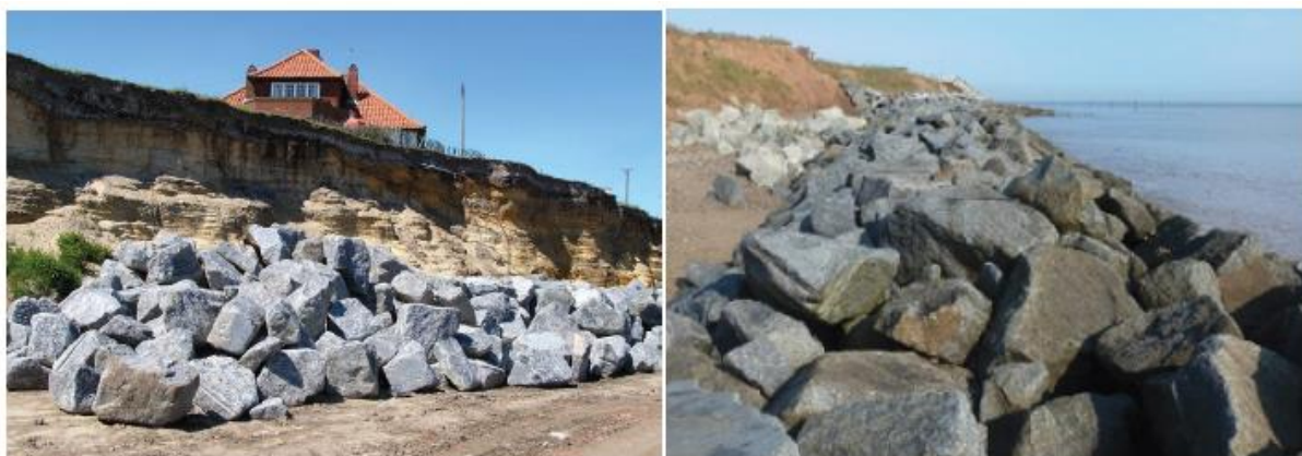
Figure 5-1: Example photographs of rock revetments in front of steep cliffs
