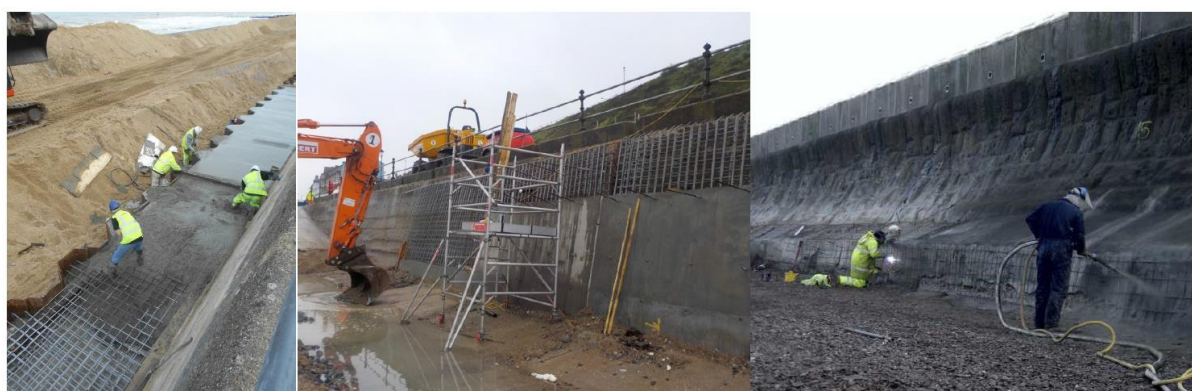
Figure 5-6: Photograph examples of re-facing seawall defences
