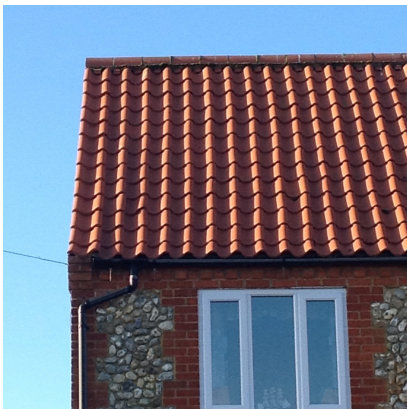
Steep pitched roof with norfolk red pantiles
