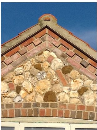
Gable with mortar verges and red brick detailing
