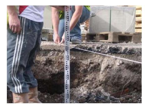
Photograph 6: Depth check of inert cover within rear gardens. Taut string line spans across excavation.
