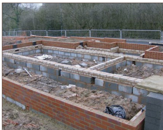
Figure A4.34 Open void >300mm deep, good ventilation through internal sleeper walls (courtesy Smith Grant)
