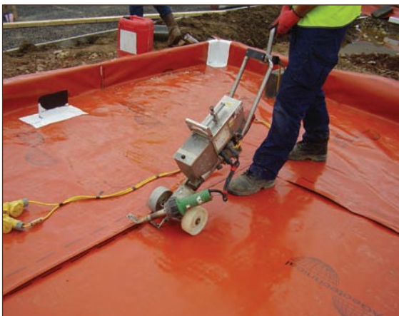
Figure A4.31 Extrusion welding (courtesy PAGeotechnical Ltd)
