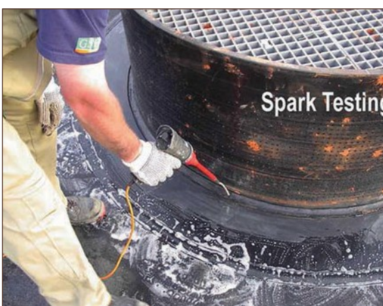
Figure A4.45 Spark testing (courtesy GSE Environmental)
