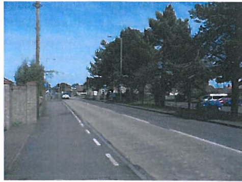
View northwards along the A149 to the Downs Road junction
