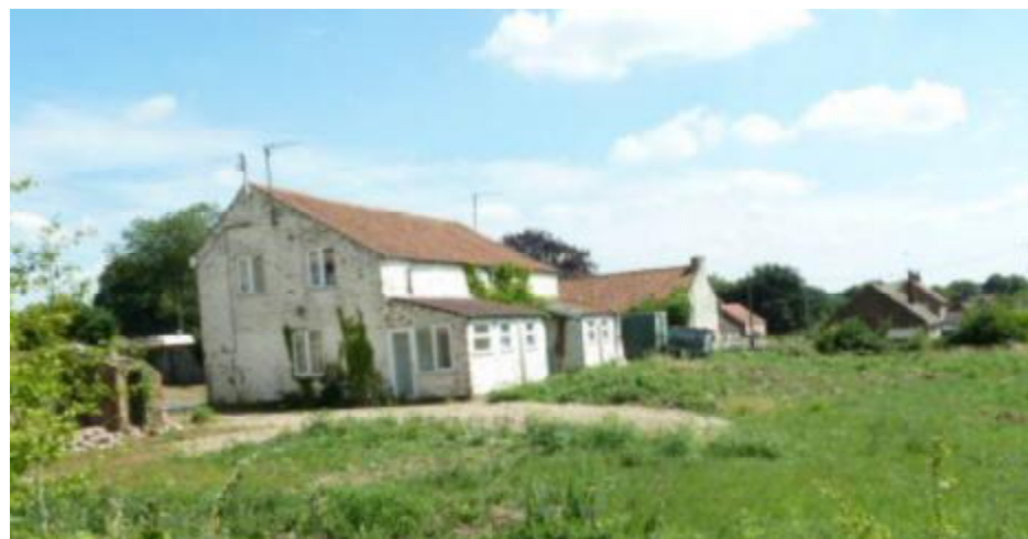
Mid twentieth century rear lean-to extensions (Photograph supplied by P. Grange)
