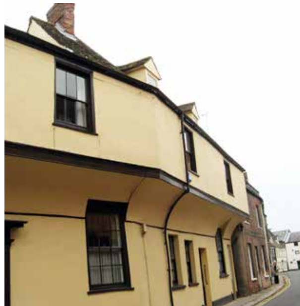
Nos. 1 and 2 Nelson Street
