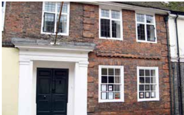
Nos. 11 and 13 Nelson Street
