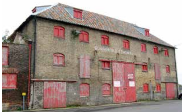
The Sommerfeld and Thomas Warehouse, South Quay
