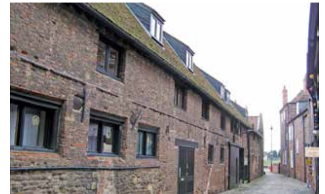
Early brickwork in King's Staithe Lane
