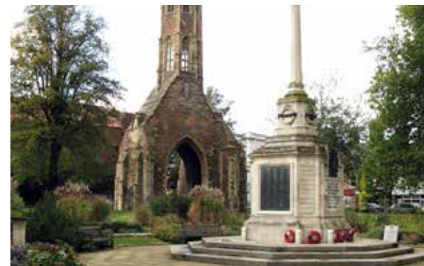
Greyfriars Tower and the War Memorial, Tower Gardens
