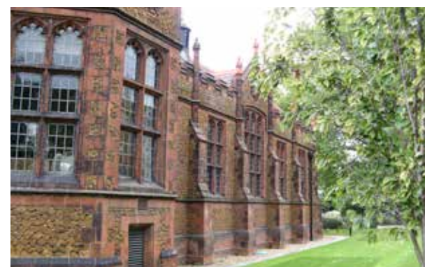
Detail of the Carnegie Library facing London Road
