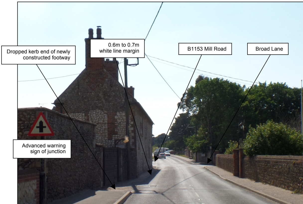
Photo 3: A149 Looking West Towards B1153/A149/Broad Lane Junction
