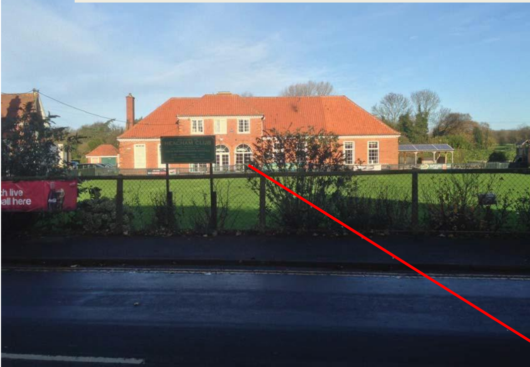
J.47 Heacham Sports and Social Club, Station Road (approx. 900m from the site)
