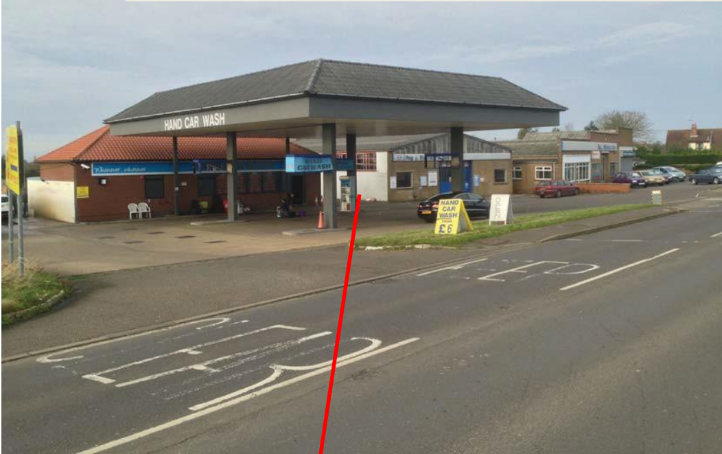
J.60 Hand Car Wash, Lynn Road (approx. 150m north of the site). New footpath will improve accessibility to existing and new residents by walking and cycling.
