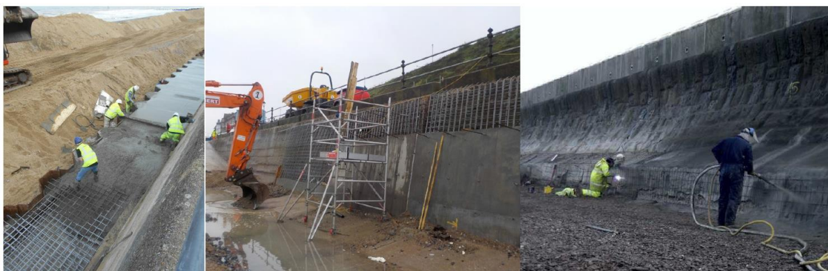
Figure 5-6: Photograph examples of re-facing seawall defences
