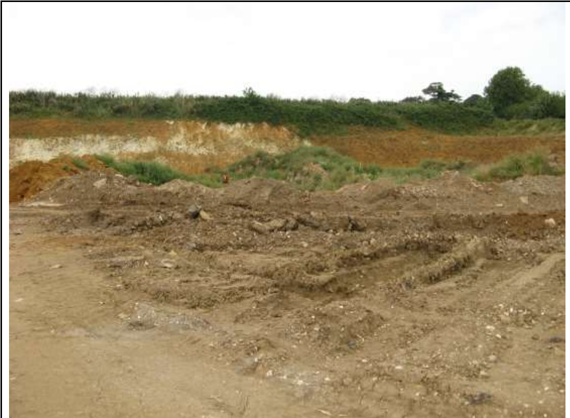
Photograph 3. Landfilled area not restored
