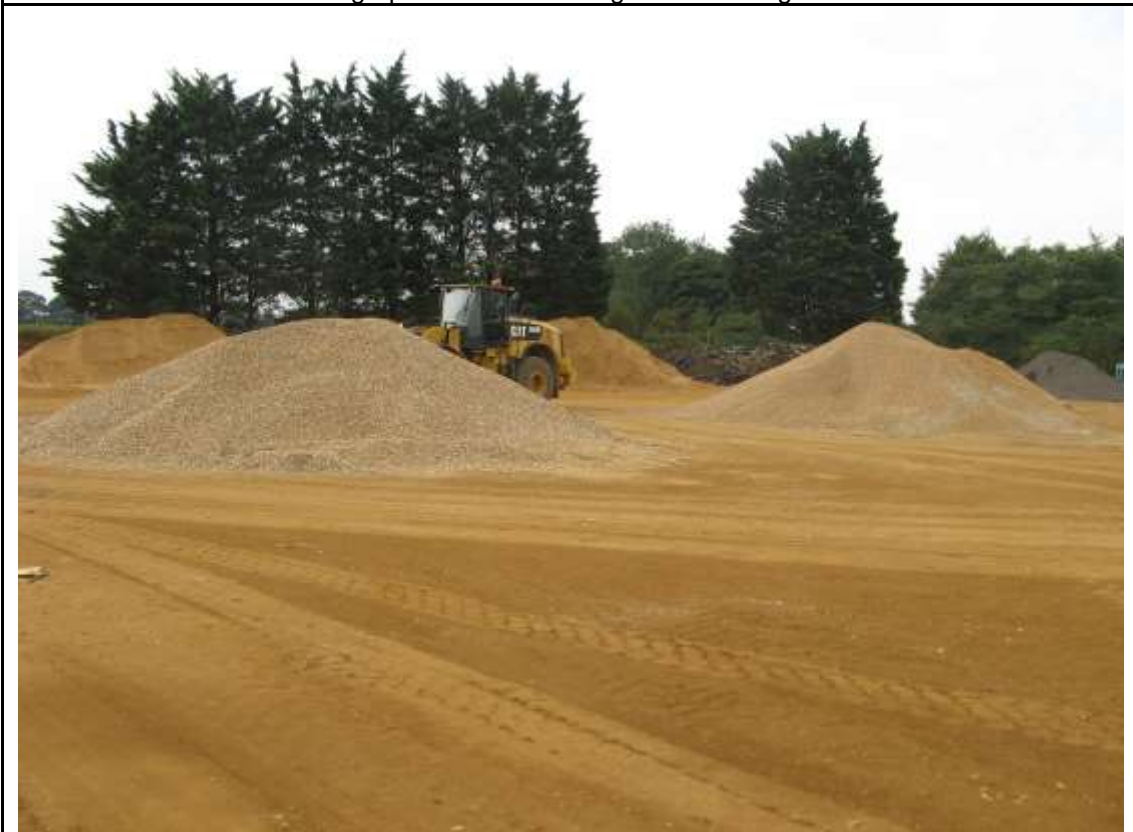
Photograph 2. Mineral storage area looking south
