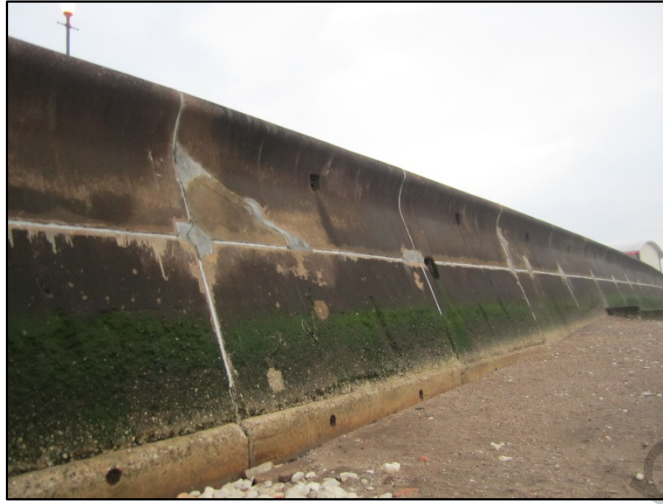
Figure 3: Photograph of recent patch repairs on seawall in Section G
