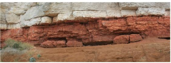
Other features present on the face which may be having an adverse effect on stability of the cliff are associated with drainage. There are numerous pipes daylighting at the crest of the cliff. The age of these pipes is not known, but it is considered likely that they are historic and that sections have broken off as the cliffs have failed around them, possibly as a result of poor joints / leakage.
