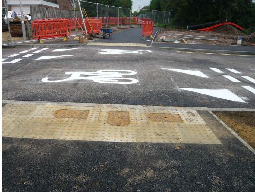
Spencer Road Crossing
