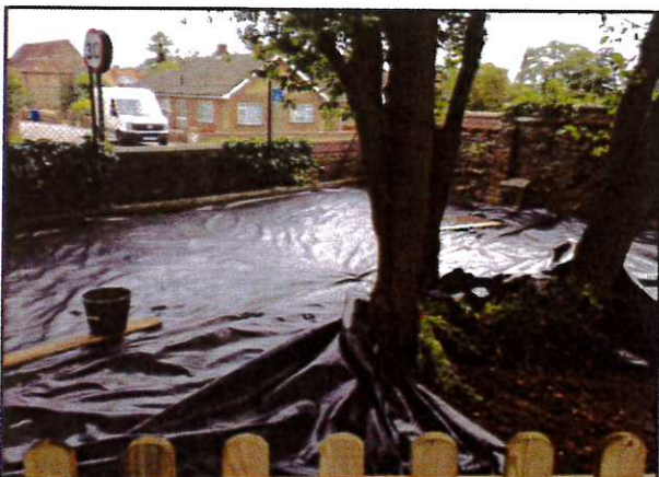
Work in progress Early June 2016
