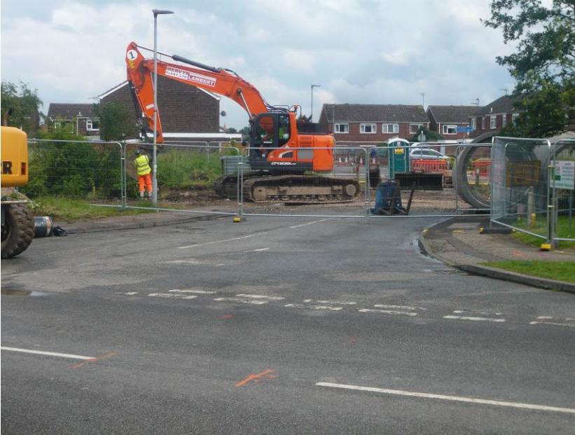
Excavation across Spencer Road
