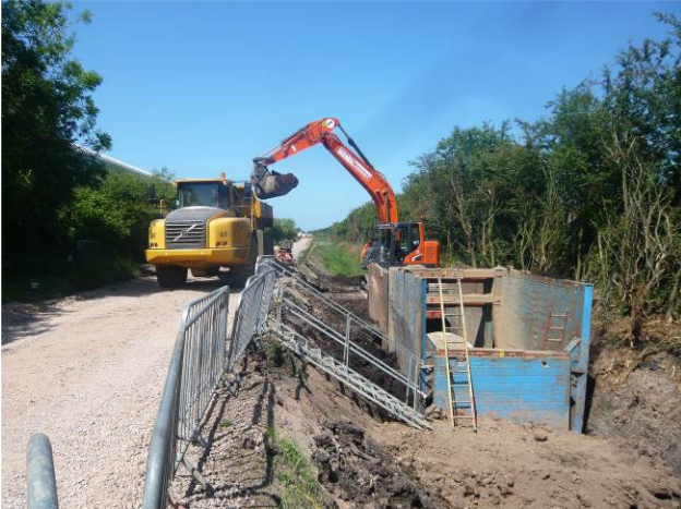
Excavating the ditch
