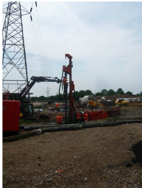
Piling rig for new road
