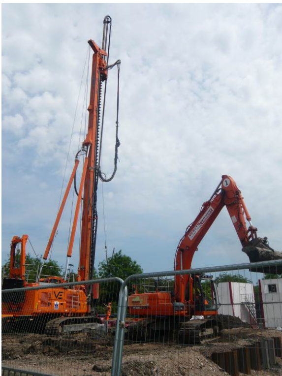
Piling rig for pumping station
