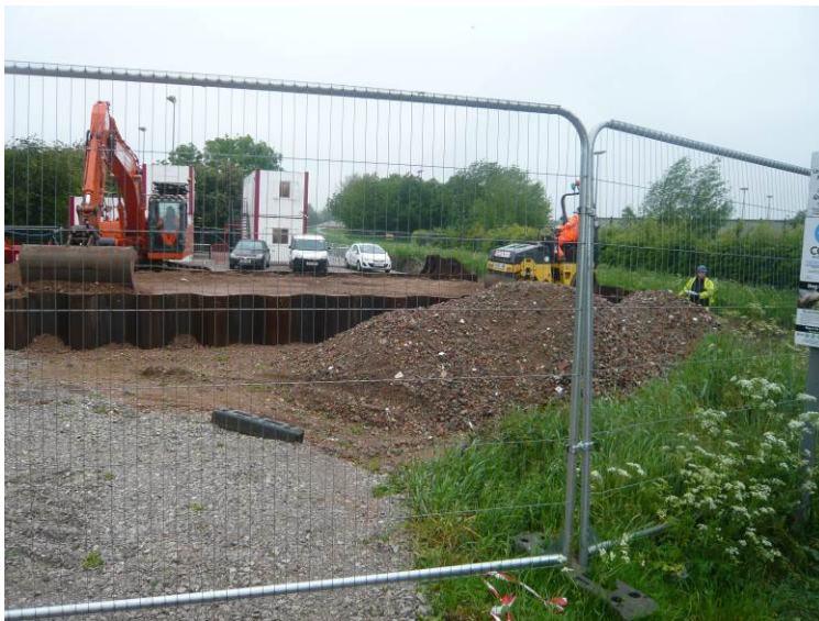
IDB pumping station works
