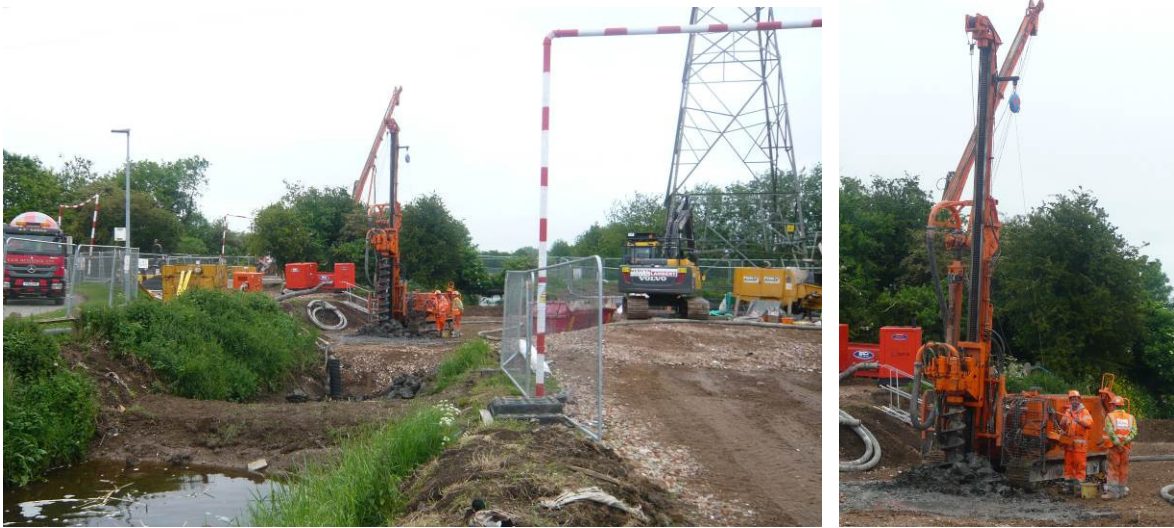
Bawsey Drain with Piling operation in progress
