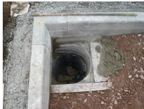
Gully under construction
