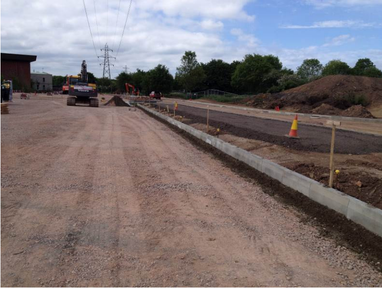
Northern car park
