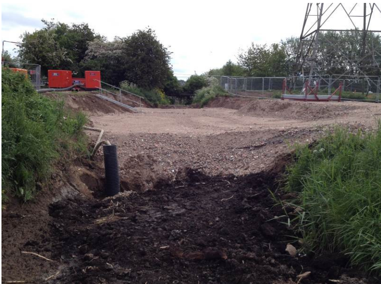
Bawsey Drain new culvert location
