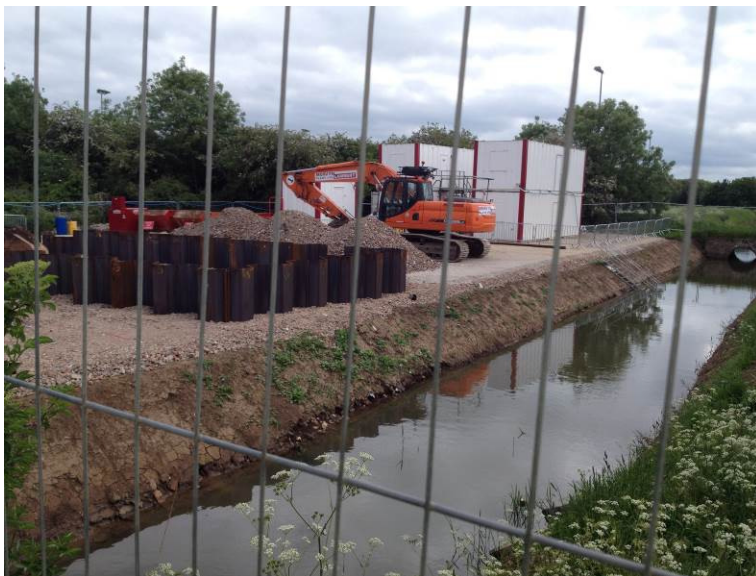
IDB pumping station works
