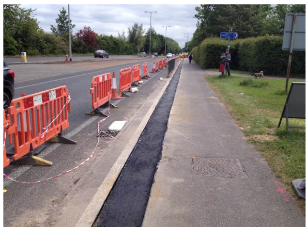
Trench for traffic signals (for detector loops)
