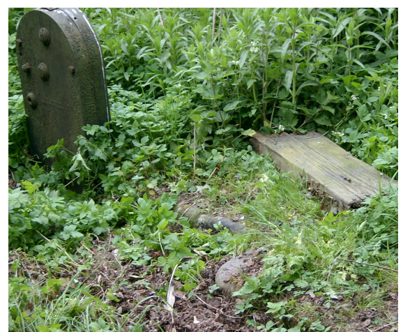
Figure 5: Photo of remains of Outwell Sluice
