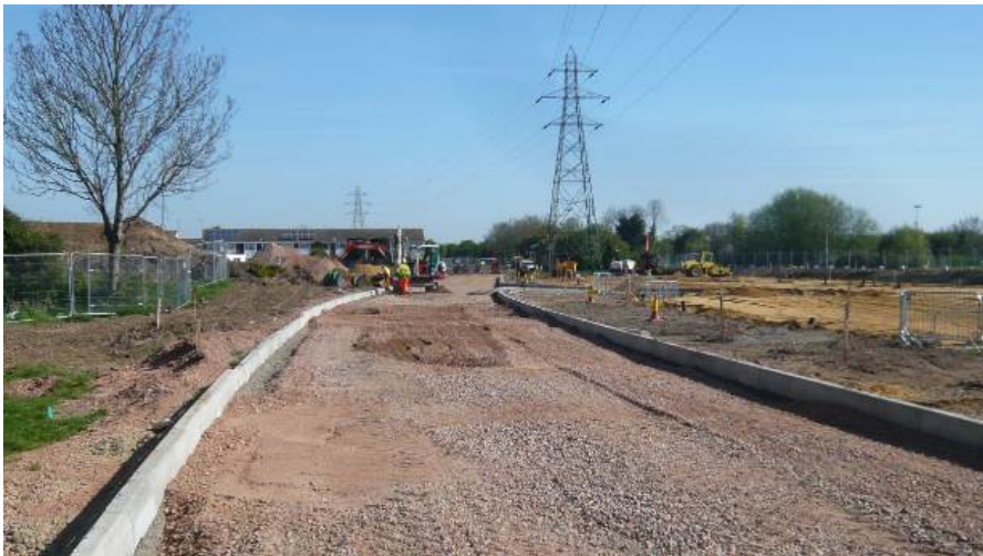
Kerbing, showing road alignment
