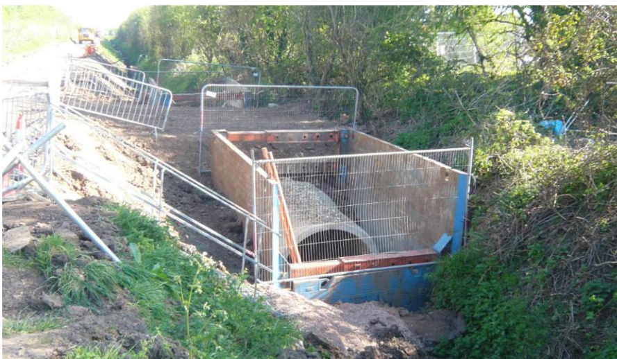
1.8m internal diameter concrete pipe
