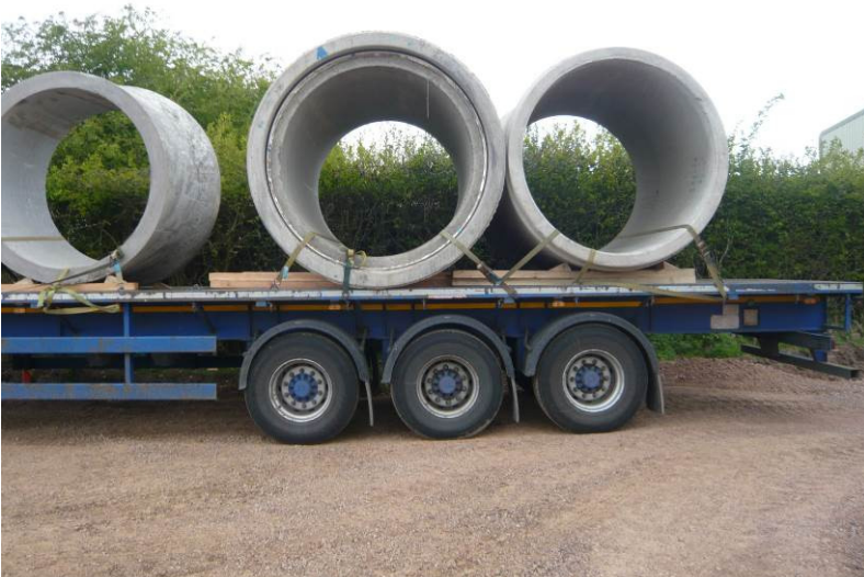
Delivery of culvert
