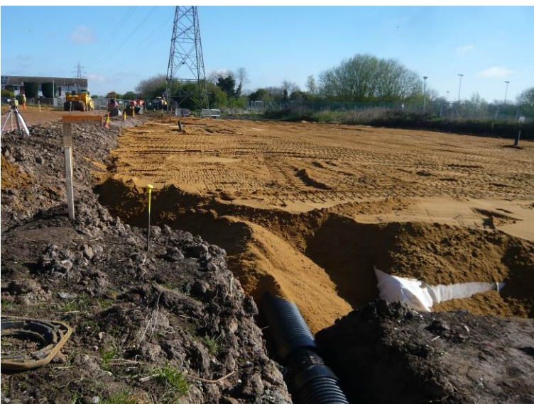
Sand fill over Aqua Cells
