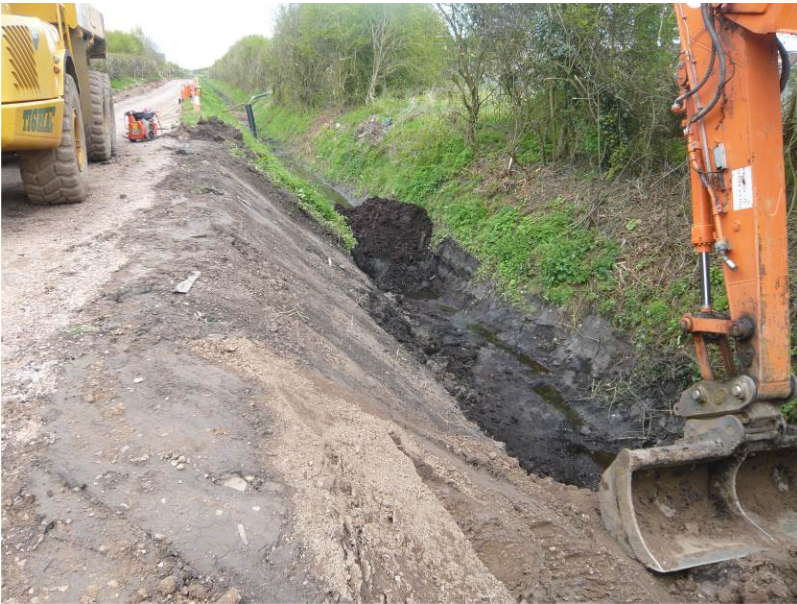
Excavator in the drain
